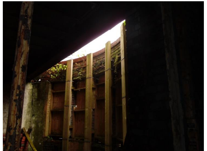
Figure 7 - Top floor at the rear of the building (internal image) - suitable bat access feature into the building
