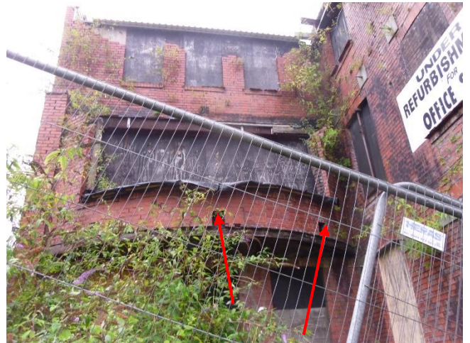
Figure 5 - Western aspect of the building. Arrows highlight suitable bat access and nesting bird features
