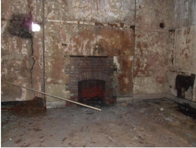
Figure 14 - Fireplace on the second floor of building
