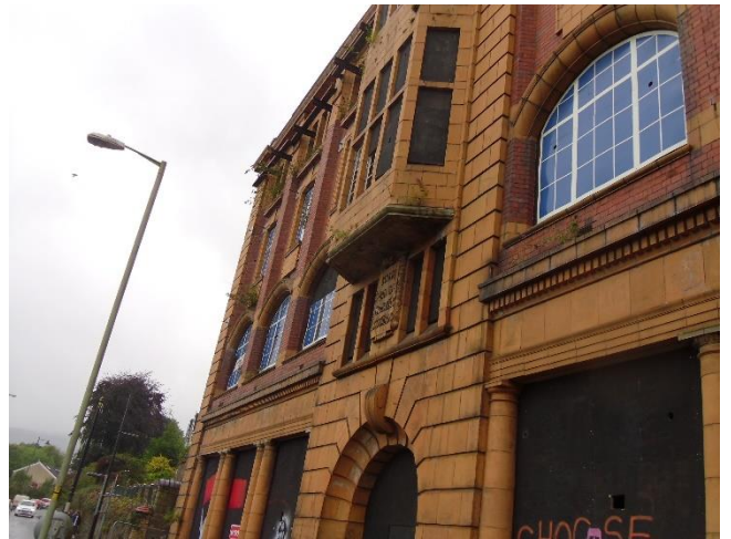
Figure 17 - Front of building
