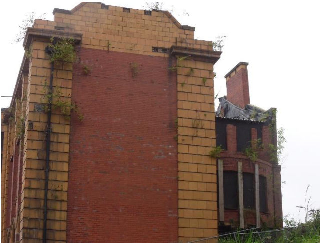
Figure 16 - Eastern aspect of building
