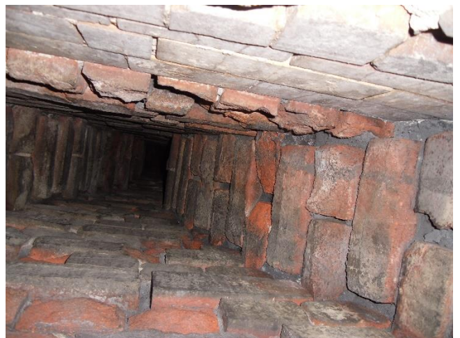
Figure 13 - Flue inside one of the many fireplaces within the building, suitable to support roosting bats
