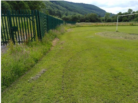
Figure 5 - Eastern fence separating the railway line access
