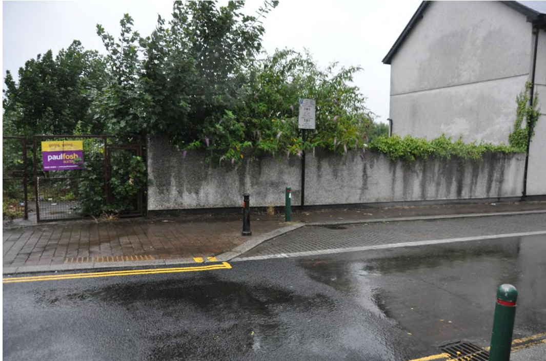
Plate 6 View of the site from Perrott street ground level
