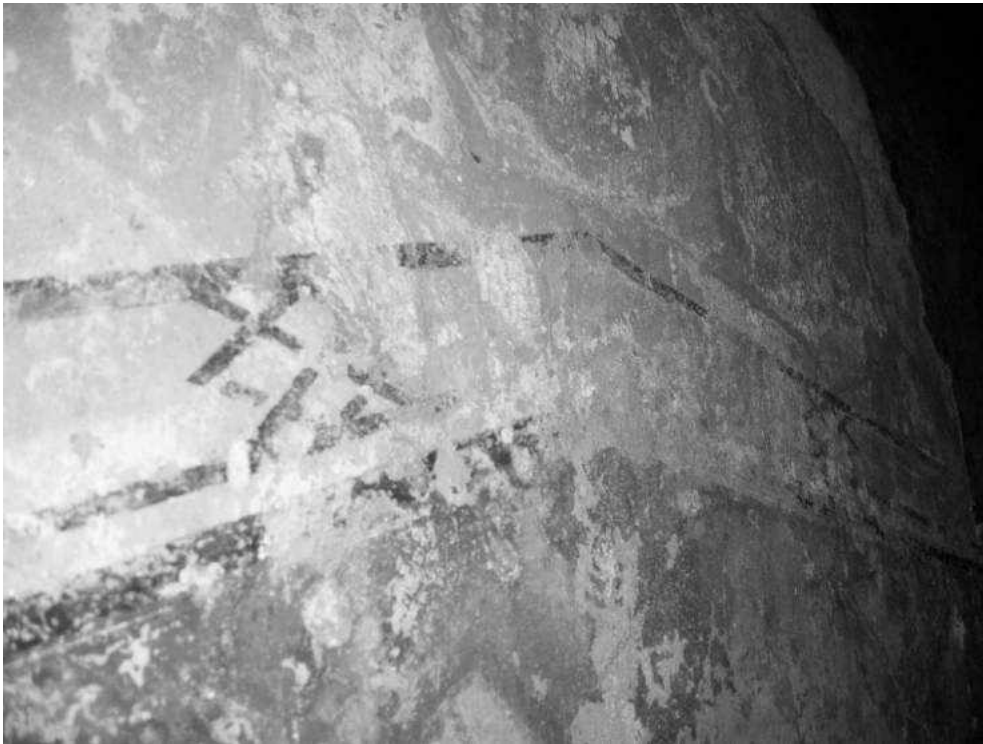
Fig 27 – stenciled decoration on staircase wall
