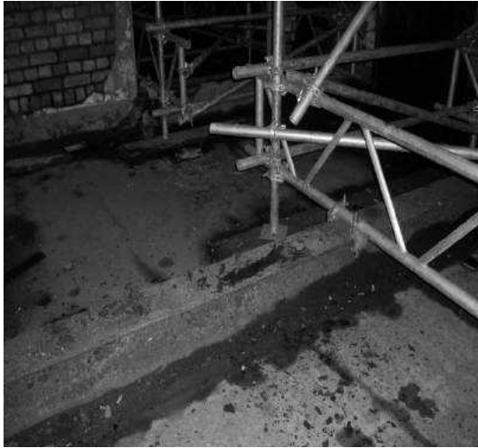
Fig 43 upstand beam on second floor
