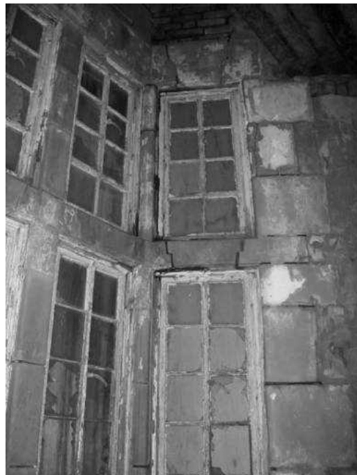
Fig 71 oriel window from landing
