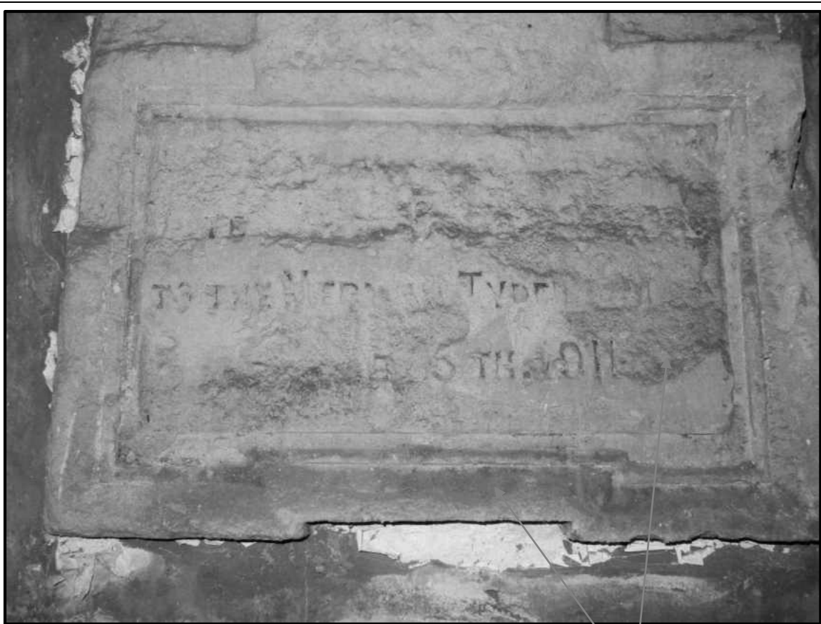
Fig 3 Plaque 1-dirty deposits, decayed stone and lost of surface.
