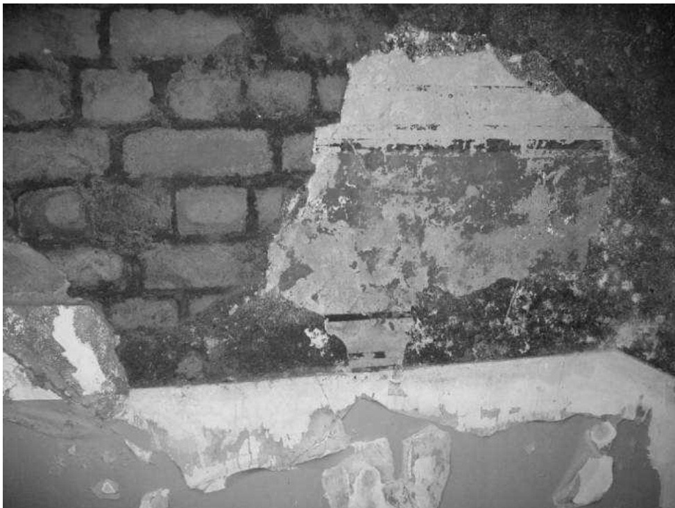
Fig 28 – stenciled decoration on staircase wall
