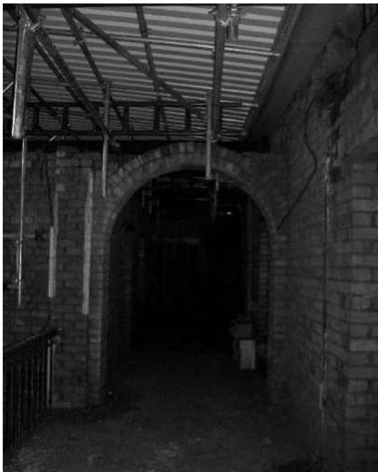
Fig 70 second floor landing
