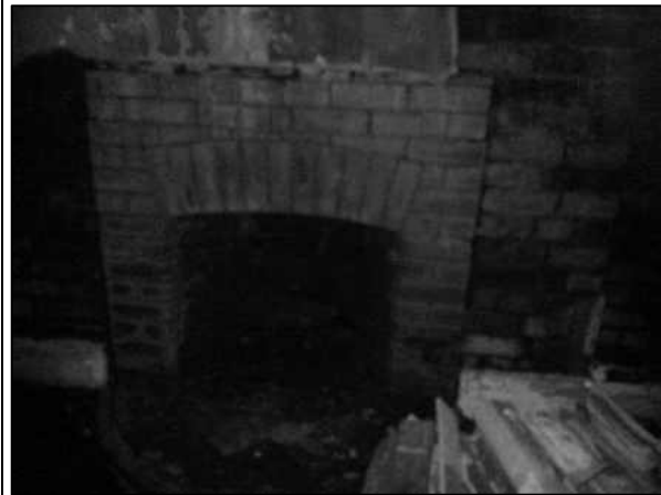
Fig 26 Another fireplace from the upper floors, simpler in style with a rounded brick hearth.
