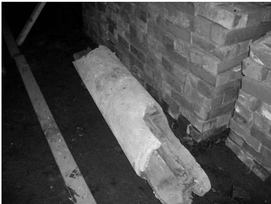
Fig 37 remains of lecture hall column
