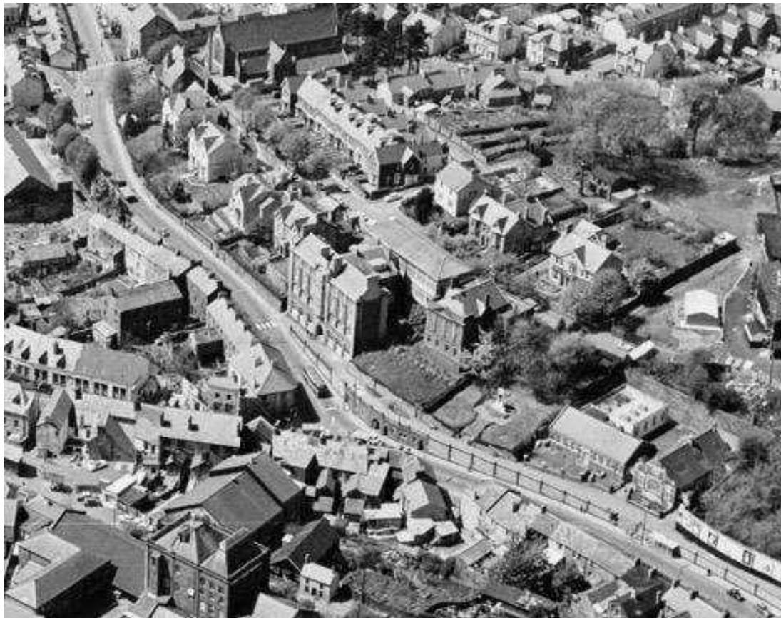
Fig 5 Aerial view 1965 showing the rear building © Davies Sutton Architects
