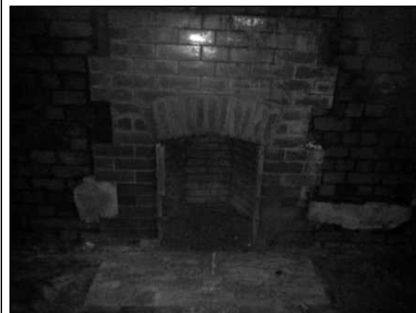
Fig 28 Upper floors- fireplace with ceramic surround and rectangular hearth.
