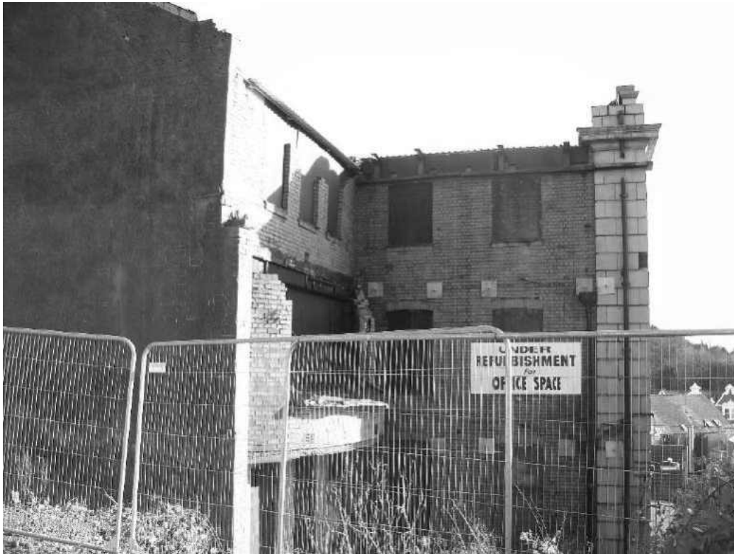
Fig 14 south-west junction of the Front and Middle Buildings
