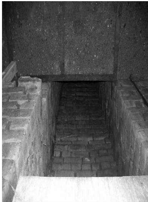
Fig 46 dumb waiter service shaft
