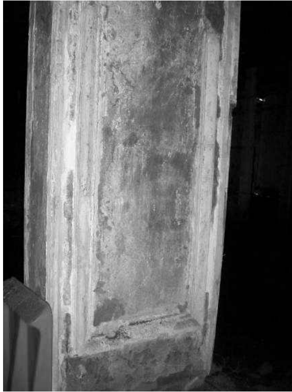
Fig 36 remains of plaster decorative detailing to lecture hall
