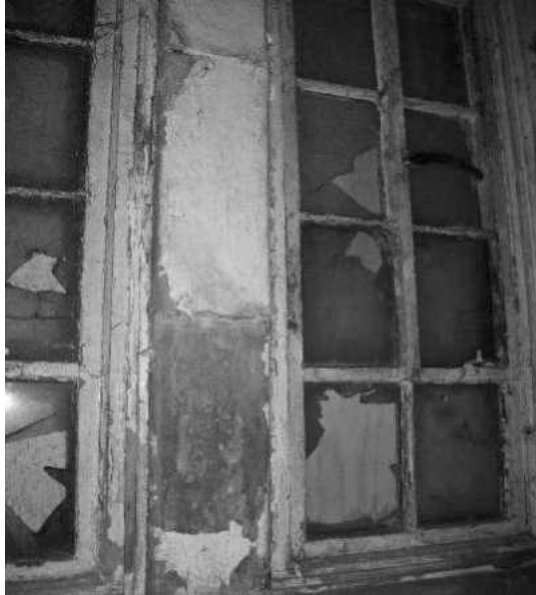
Fig 53 window frame to oriel on landing
