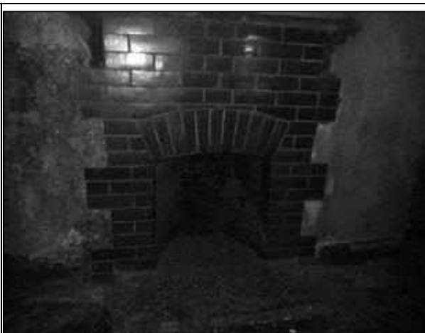
Fig 24 Another fireplace from the upper floors, very similar in style with similar brickwork hearth & back but slightly smaller.
