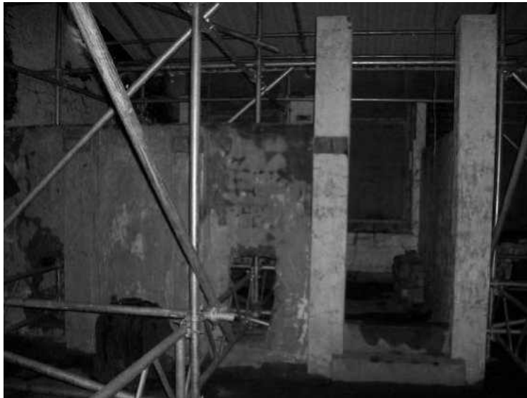
Fig 42 shower area on second floor
