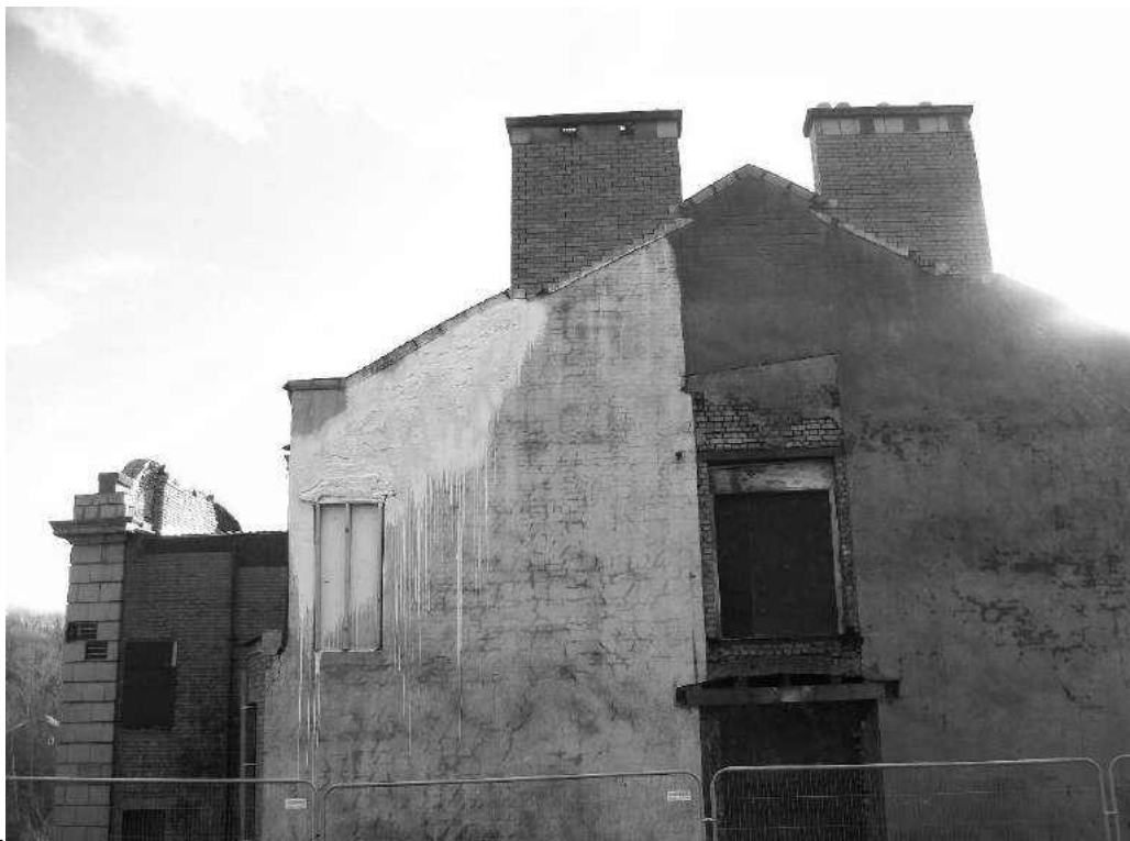
Fig 15 Middle Building gable end
