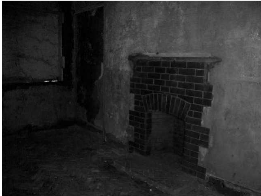
Fig 33 Fireplace in former Conversation and Smoke Room to north
