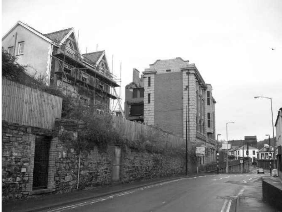
Fig 64 View from south towards YMCA
