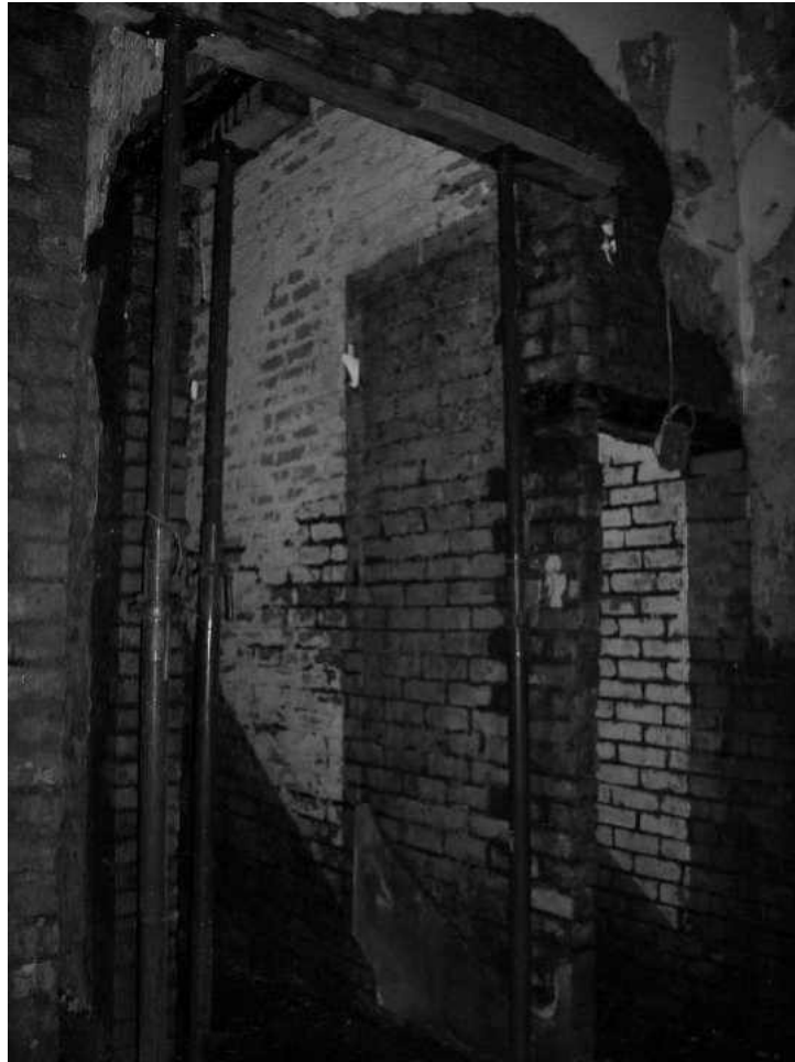
Fig 23 location of former rear stairs to south
