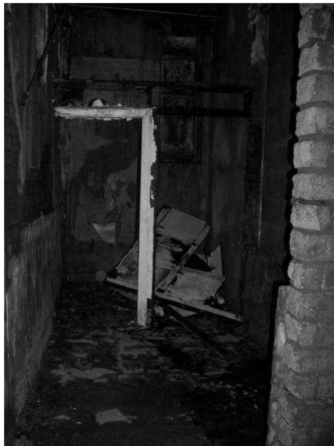
Fig 39 much altered former toilets area of first floor
