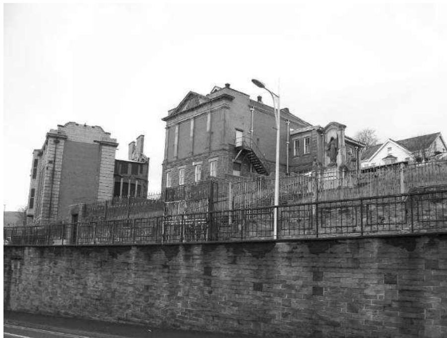
Fig 65 view from north towards YMCA (including Masonic Hall and War Memorial)
