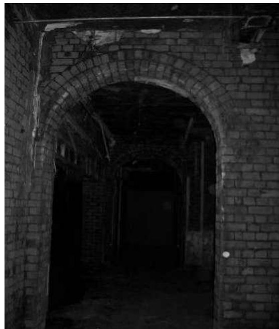
Fig 56 typical brickwork - spinal corridor
