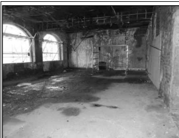
Fig 21 First floor shown prior to windows being boarded up – a fireplace aperture can be seen in the background.
