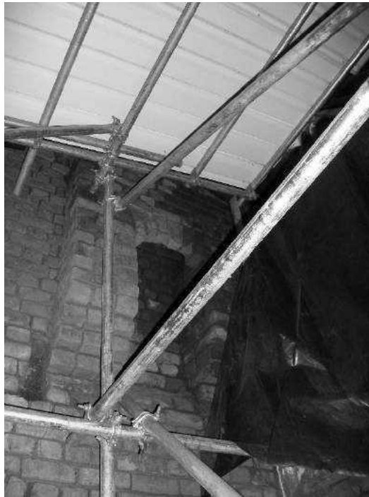
Fig 48 Third floor fireplace
