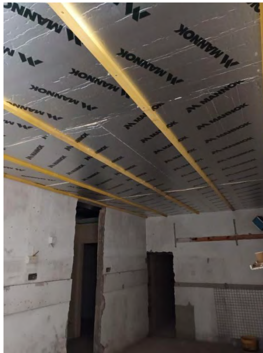
Plate 3-Room B-View of Recently Installed Ceiling Insulation Boards
