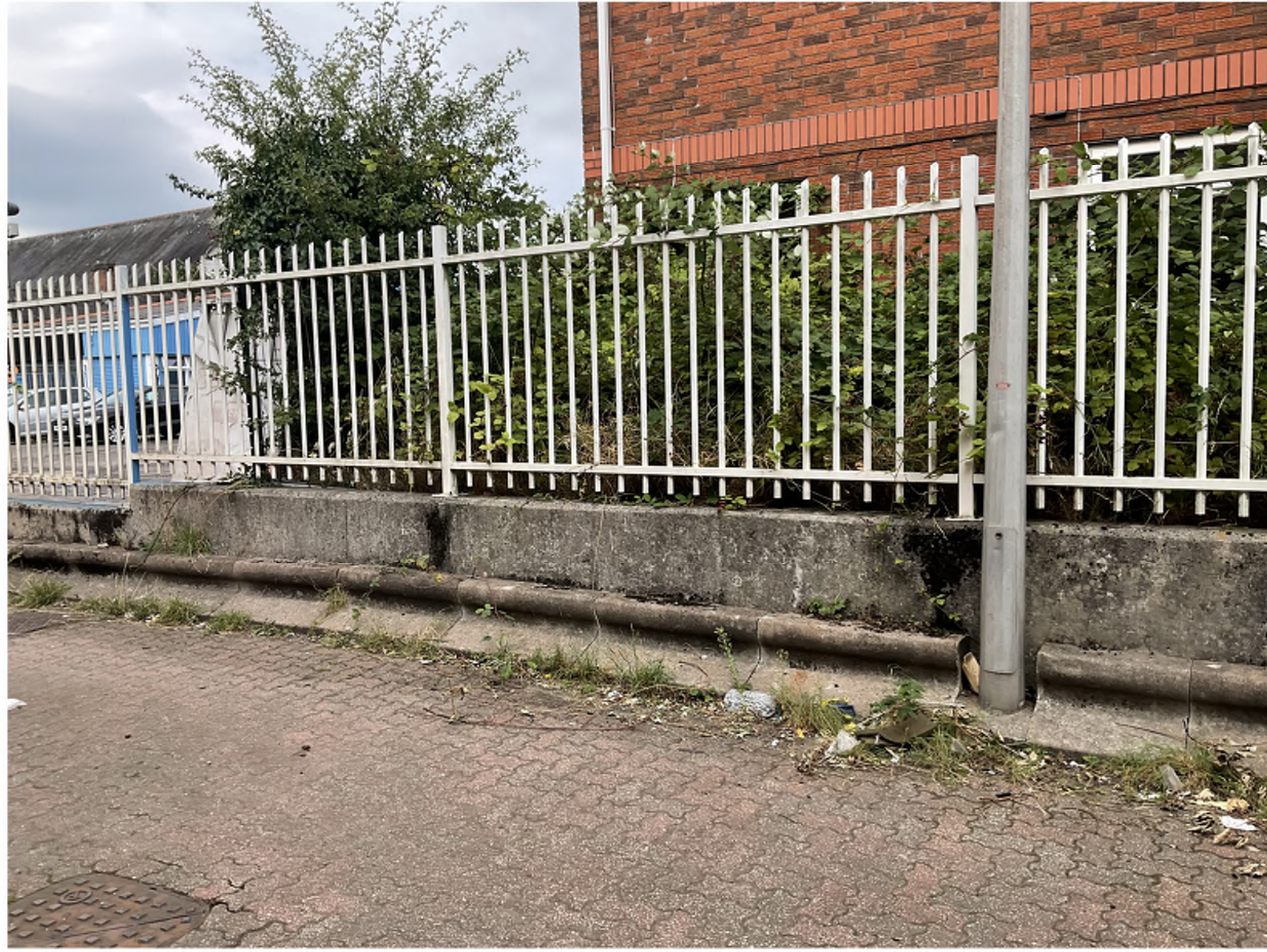
Photo 3 - Existing rear boundary railings - adjoining Fire Station
