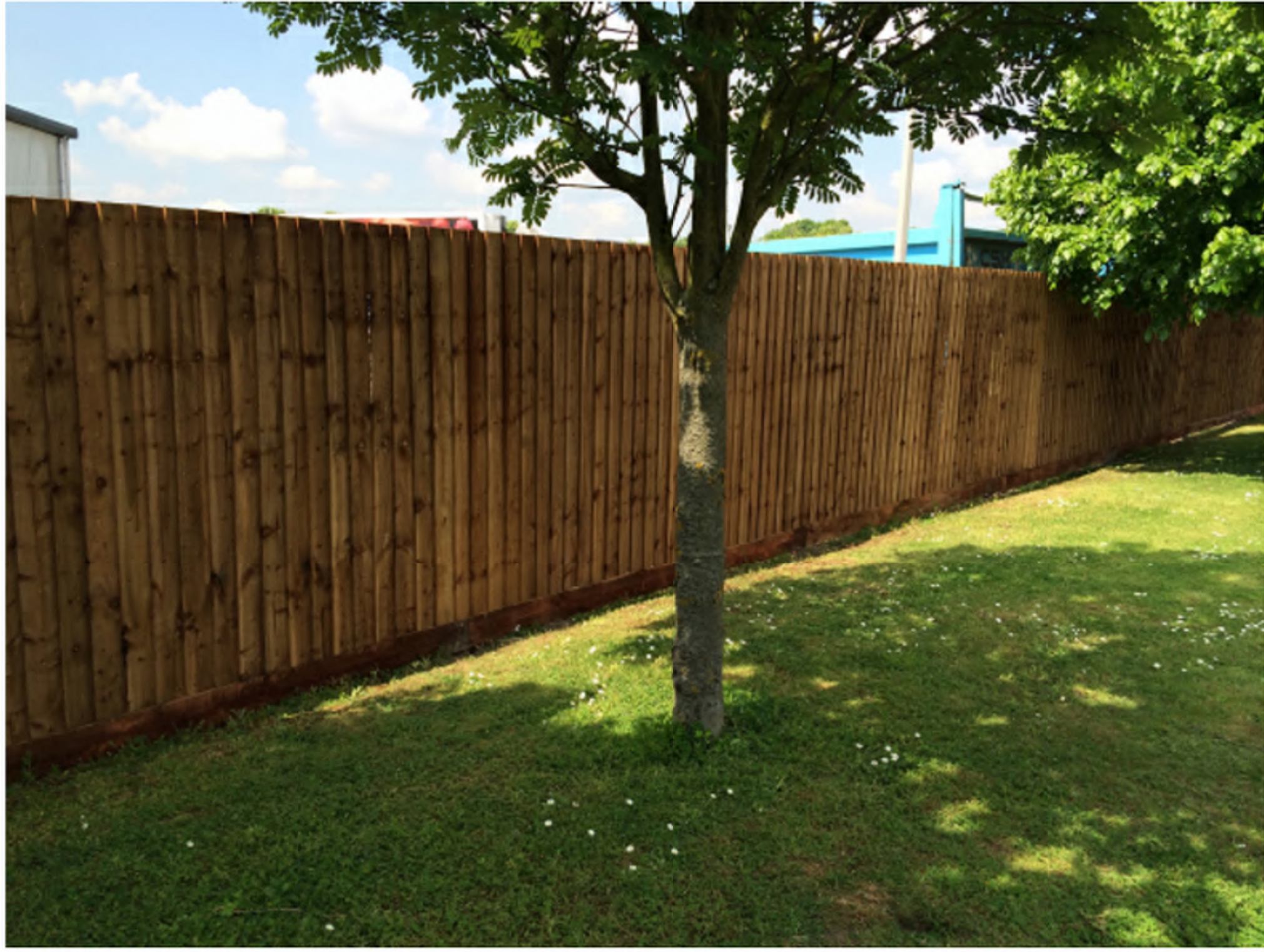
Photo 4 - Proposed specification - timber close-boarded fencing @ 2m
