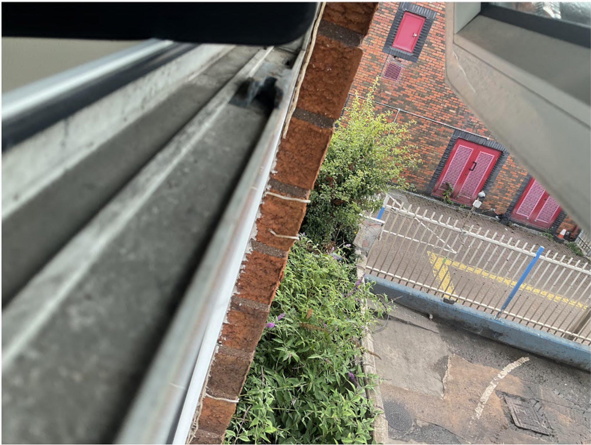
Photo 1 - Area currently overgrown - to be cleared as part of works
