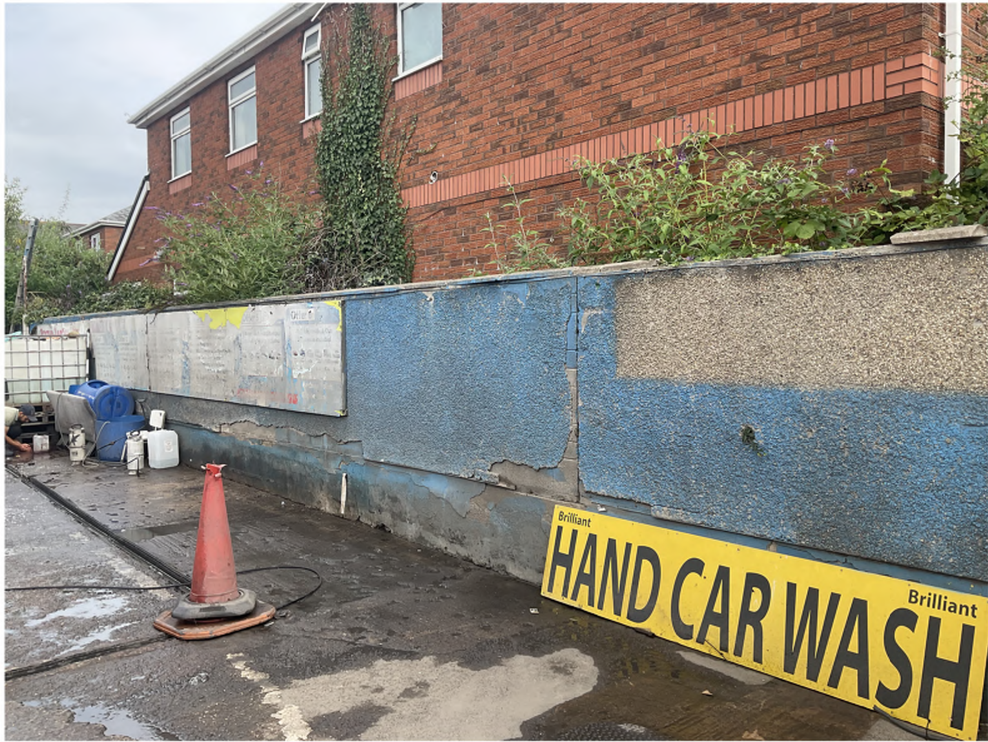
Photo 2 - Existing rear boundary wall - adjoining Car Wash
