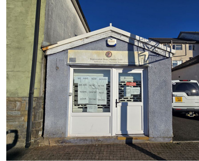
Image 3: External Front Elevation. - As taken onsite July 2025
