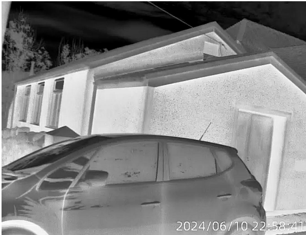
Figure 4- Thermal Guide camera view 10 th June 2024
