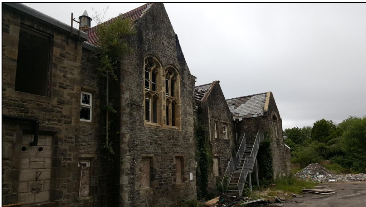
Photo 6: TN01 Derelict hospital buildings (main building)
