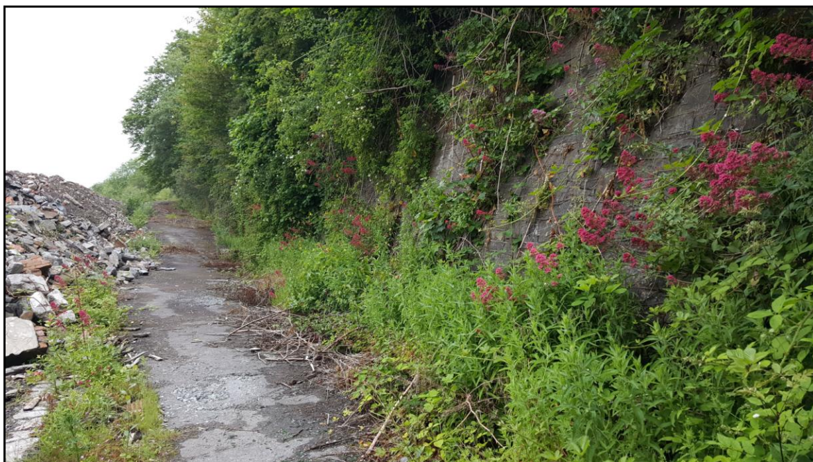
Photo 4: TN5 Eastern retaining wall
