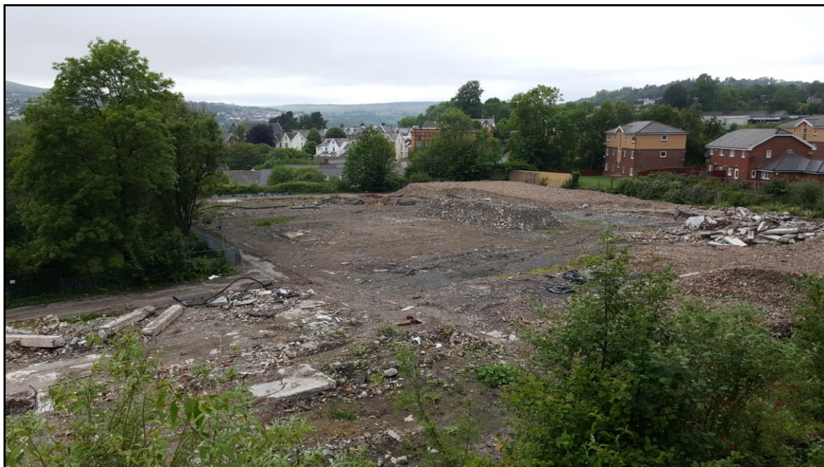
Photo 3: TN4c Overview of northern part of site
