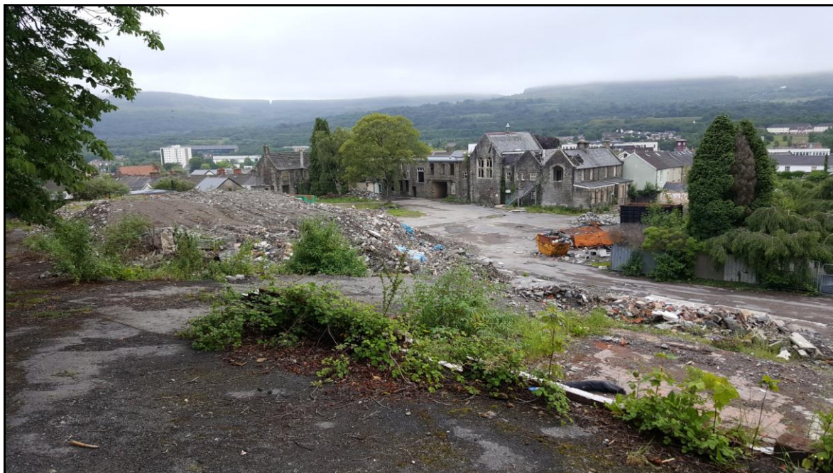
Photo 1: Overview of southern part of site showing buildings & southern TPO trees
