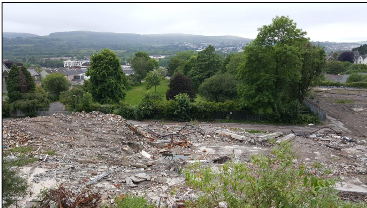
Photo 2: Overview of central part of site
