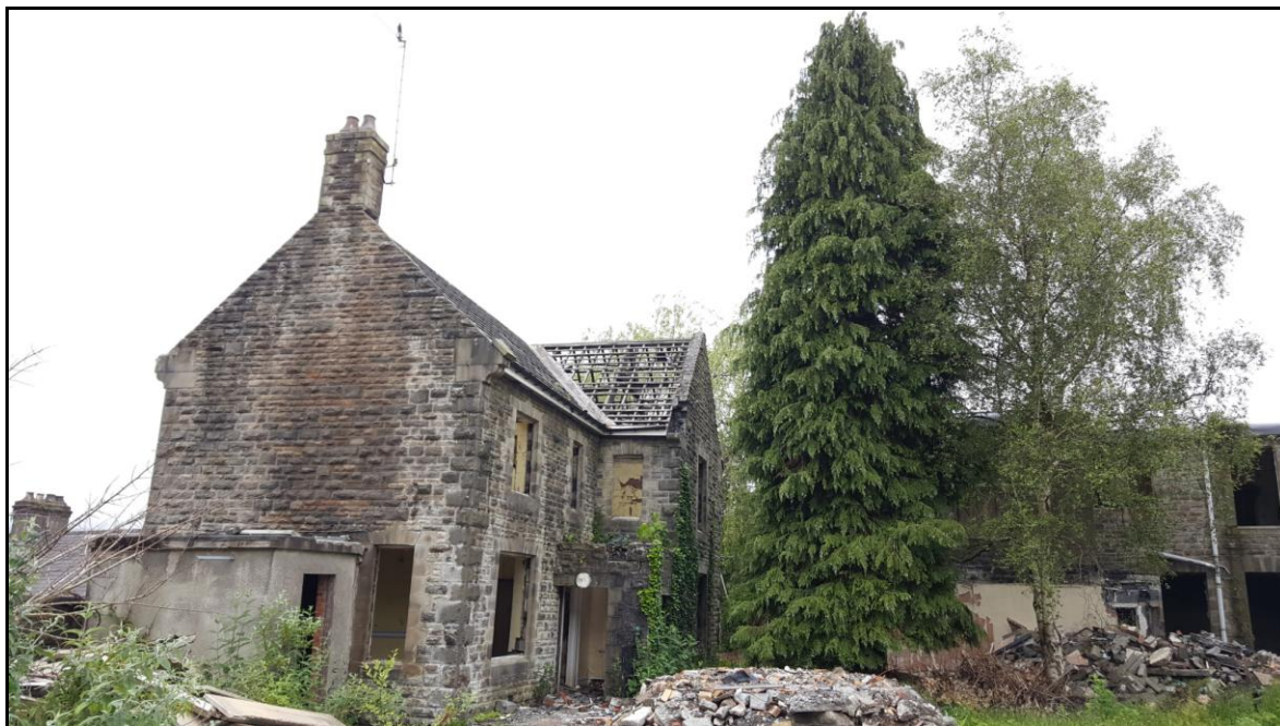
Photo 5: TN01 Derelict hospital buildings (south building)
