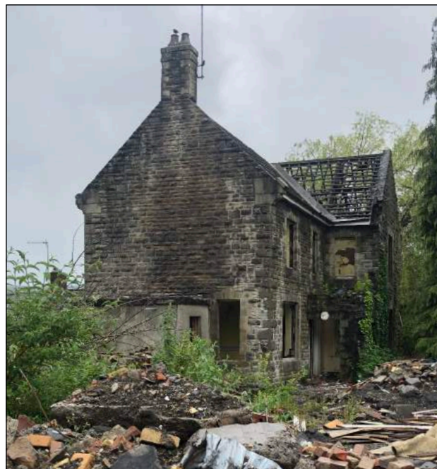
North east elevation from within the site
