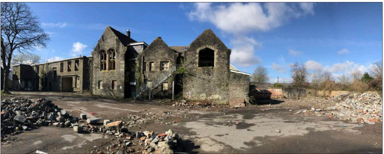
View of the rear of the listed building
