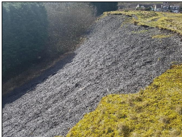
Photo 10: Exposed colliery spoil
