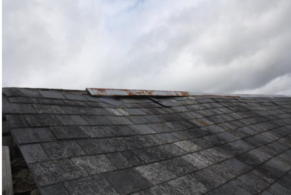
Photo 7: Gaps under fascia on northern elevation
