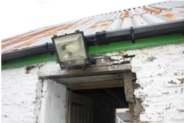
Photo 11: Gaps in stonework around door on northern elevation
