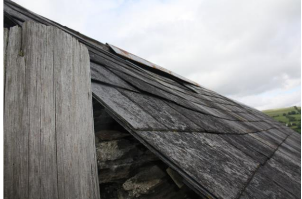
Photo 8: Gap under ridge at eastern gable end
