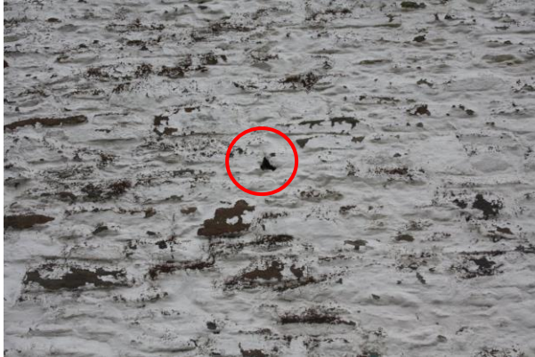
Photo 11: Gaps in stonework around door on northern elevation
