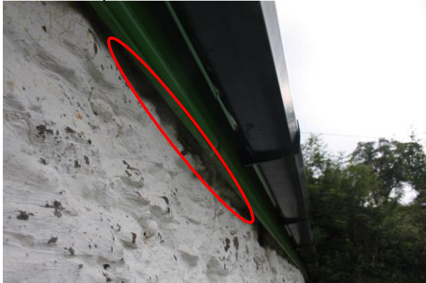
Photo 9: Example of crevices in external stonework
