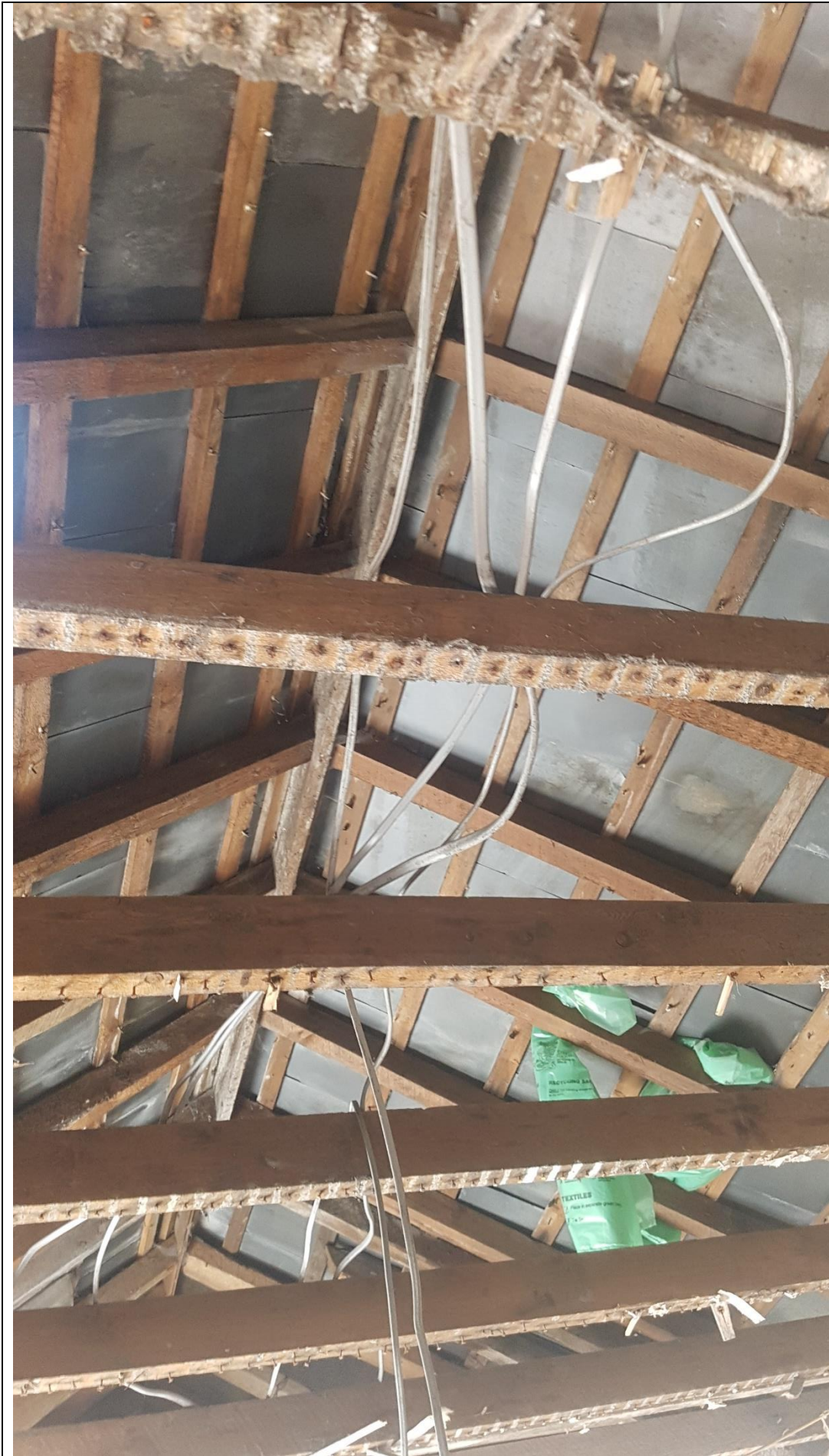
Photo 5. Underside of the roof covering
