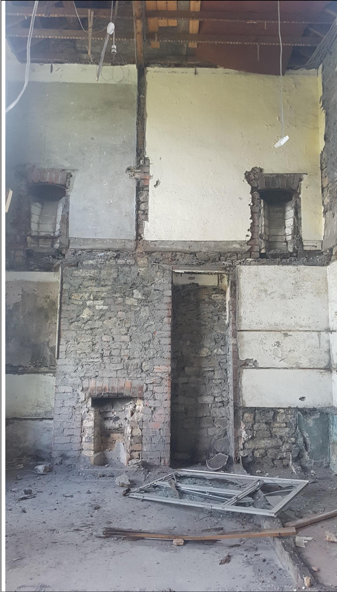
Photo 8. Ground and former first floor interior
