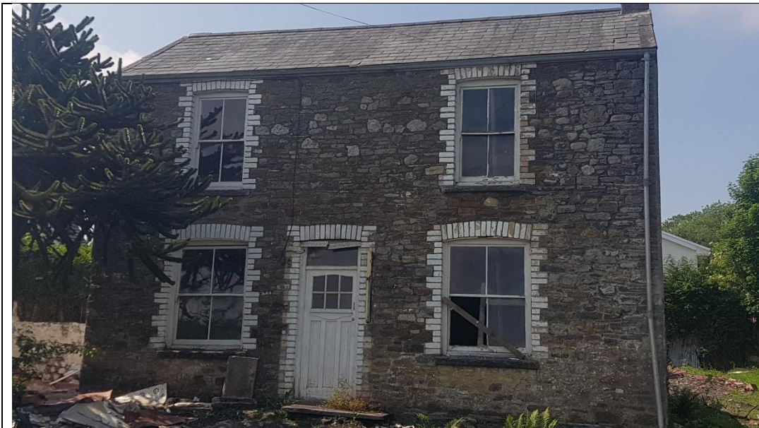
Photo 1. Front elevation of Waunfach House (north). Windowpane opened for access but usually covered by board.
