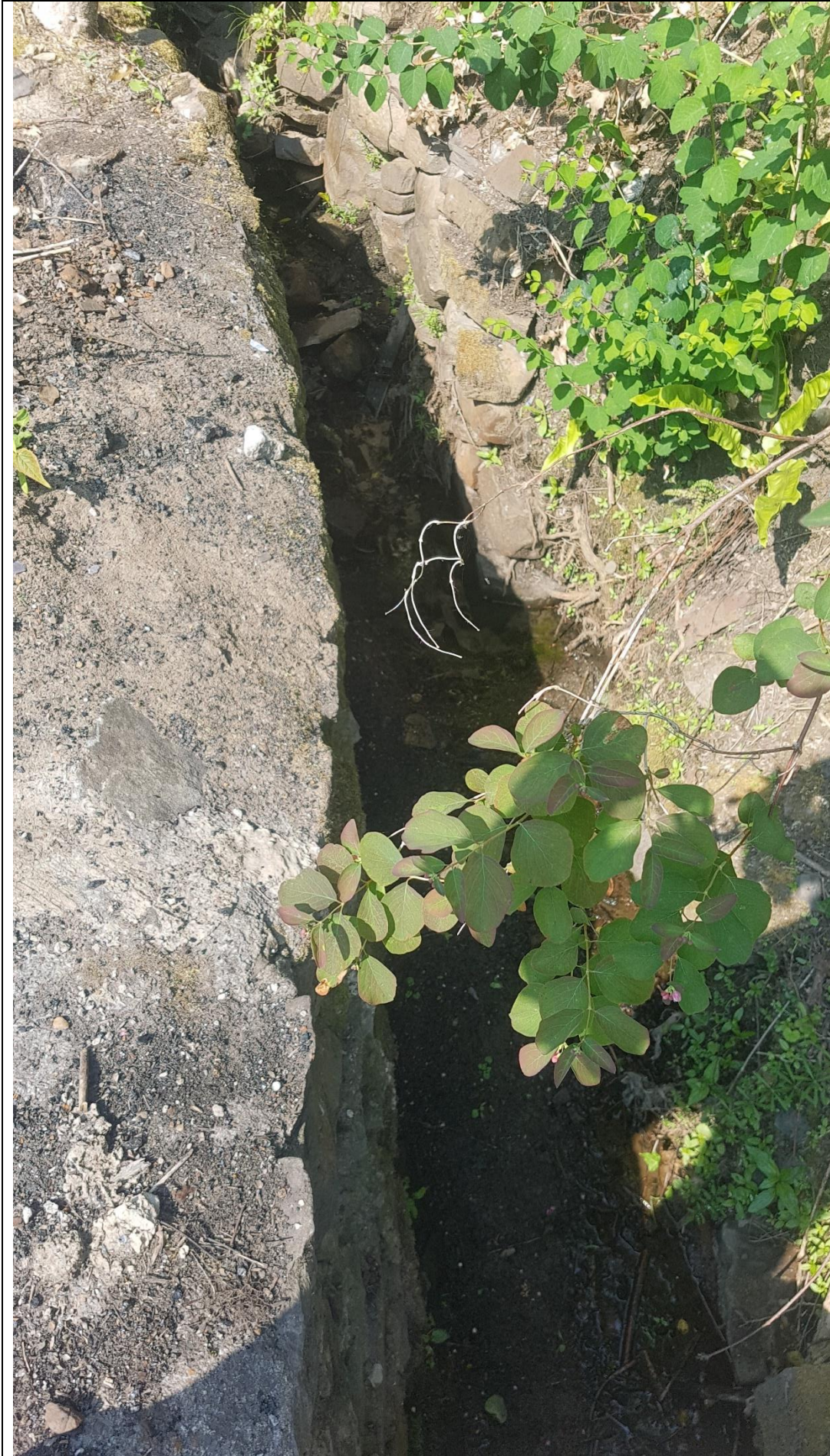
Photo 9. Unnamed watercourse running through the corner of the site before it is culverted
