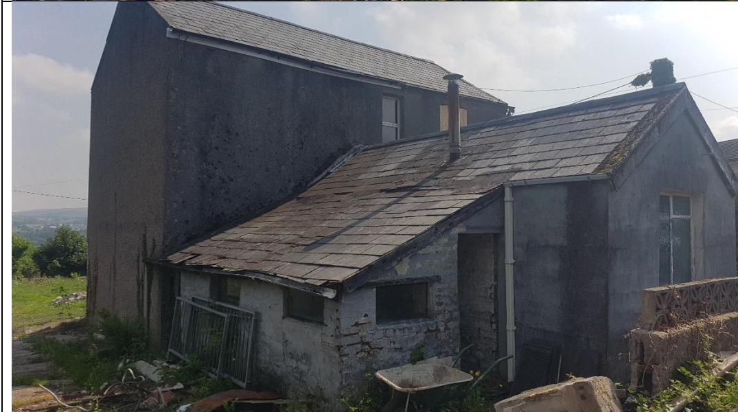
Photo 2. Side and rear elevations showing extension (west and south)
