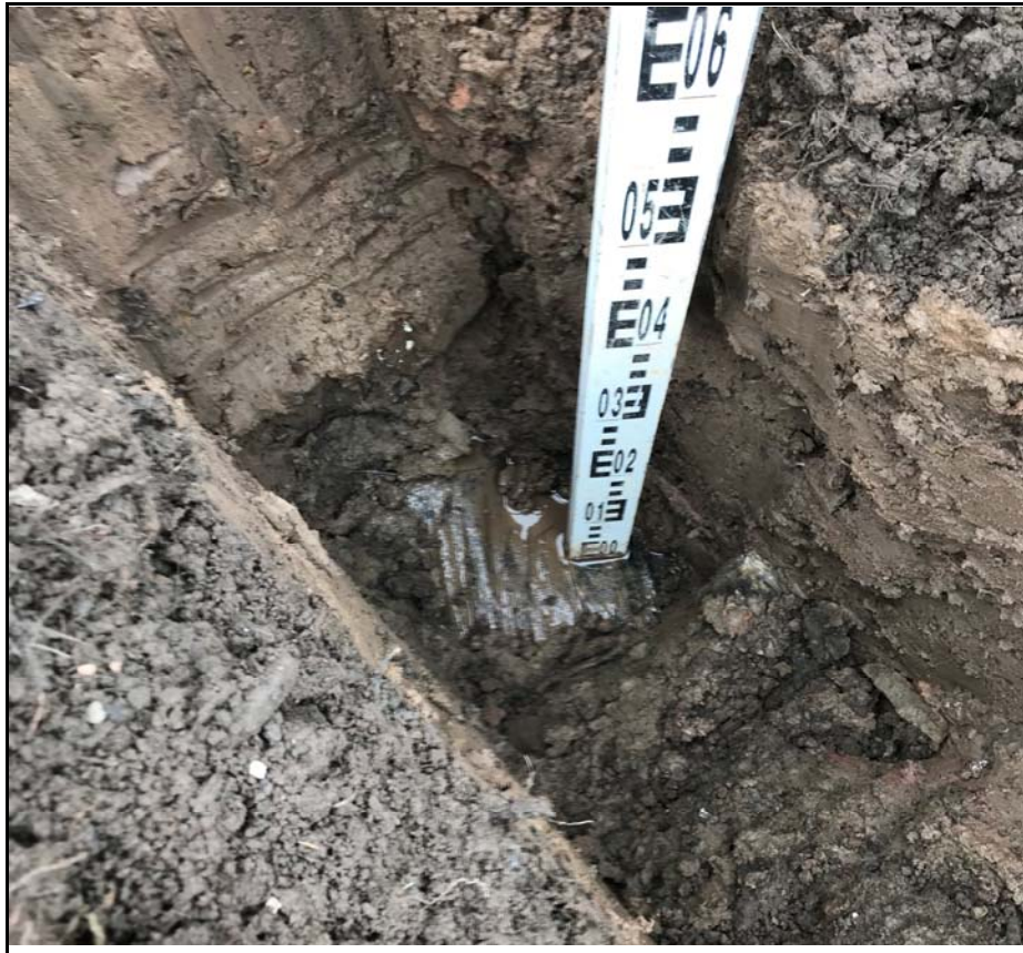
Plot 146 Showing Membrane at Base of Soils
