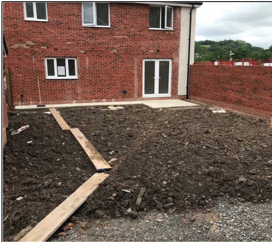
Plot 147 Depth Check Excavation Pit
