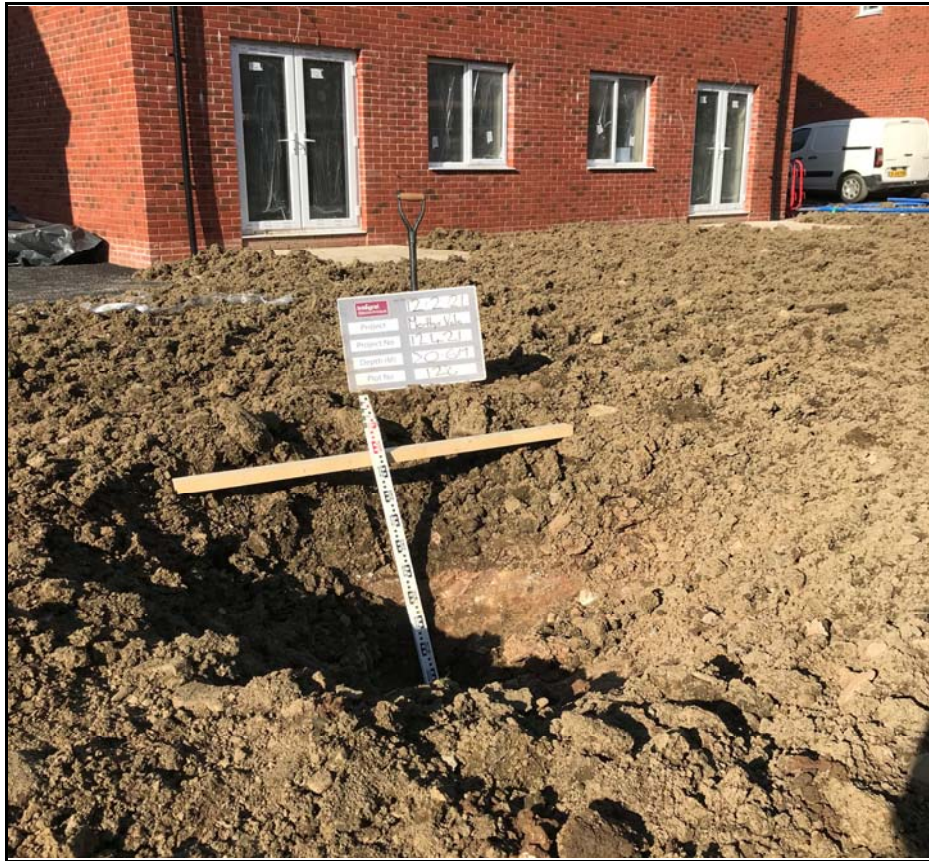
Plot 126 Showing Capping Depth Check
