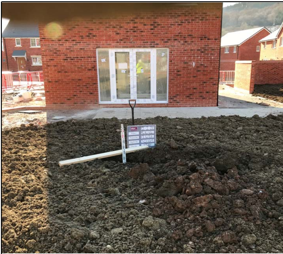
Plot 128 Showing Capping Depth Check
