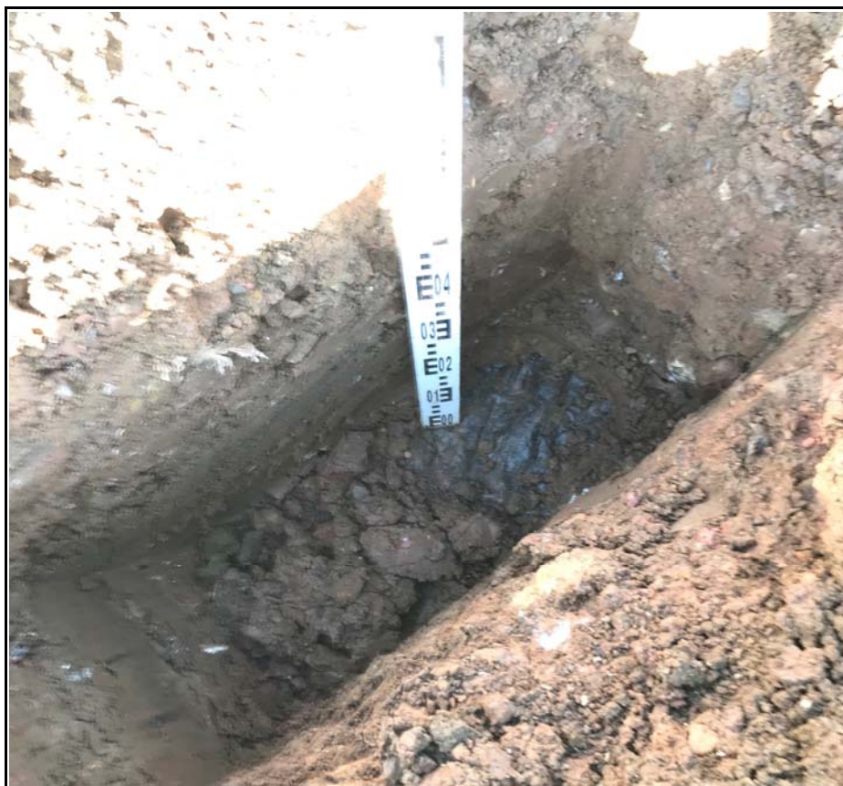
Plot 135 Showing Membrane at Base of Soils
