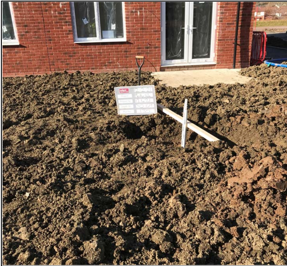
Plot 135 Showing Capping Depth Check
