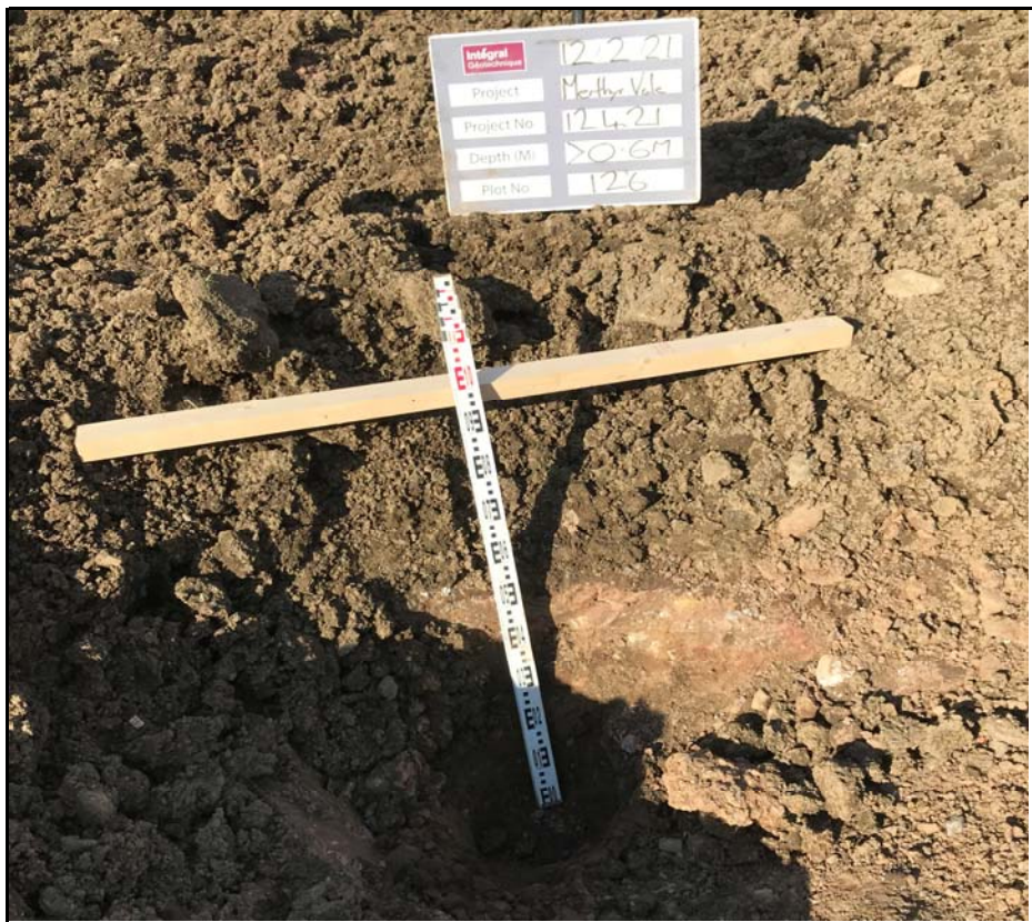
Plot 126 Showing Excavation Trial Pit
