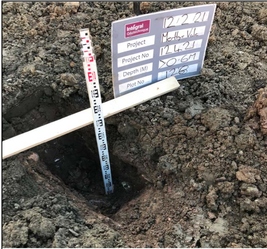
Plot 128 Showing Excavation Trial Pit
