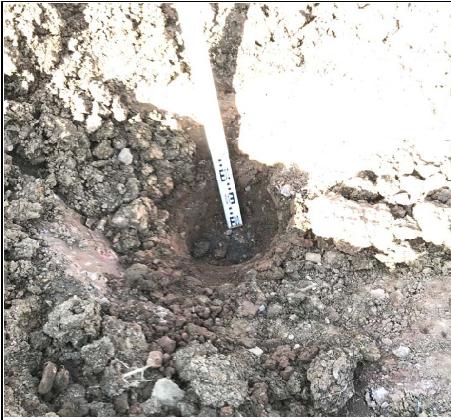
Plot 126 Showing Membrane At Base of Soils
