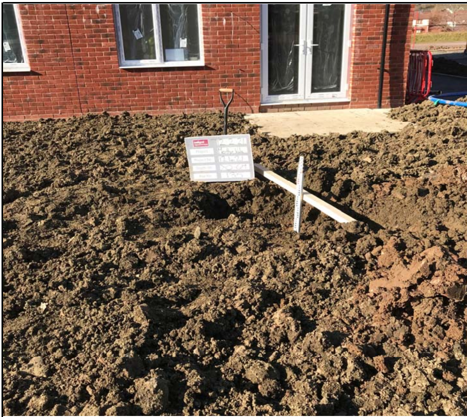
Plot 135 Excavation Trial Pit
