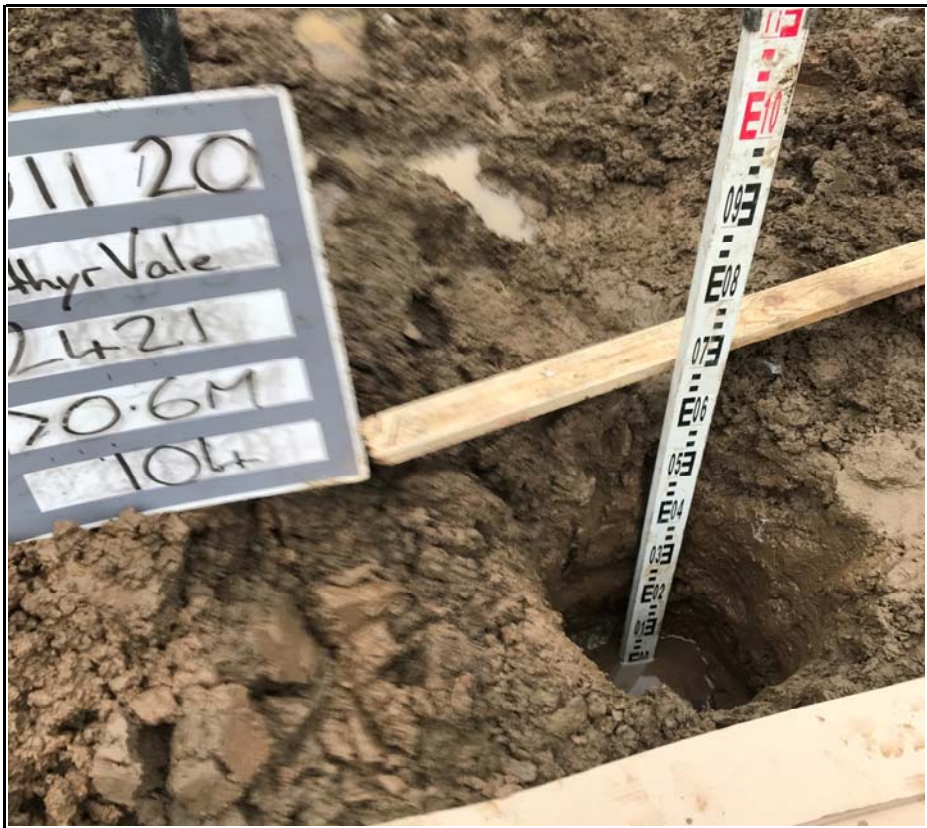
Plot 104 Excavation Trial Pit
