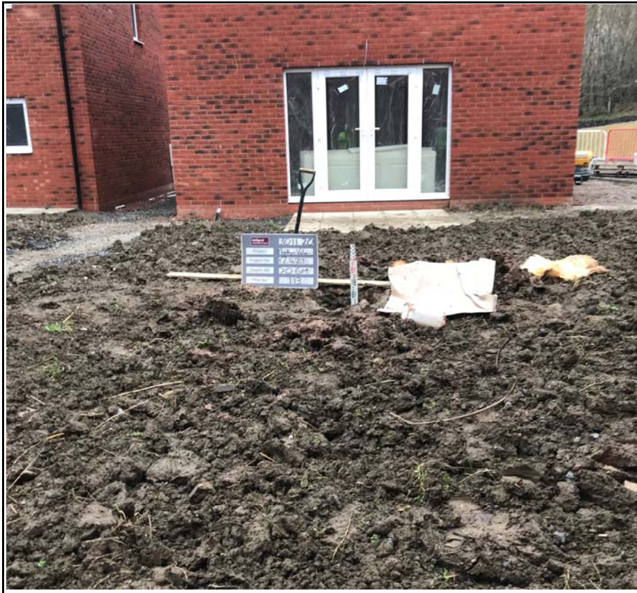
Plot 113 Showing Capping Depth Check
