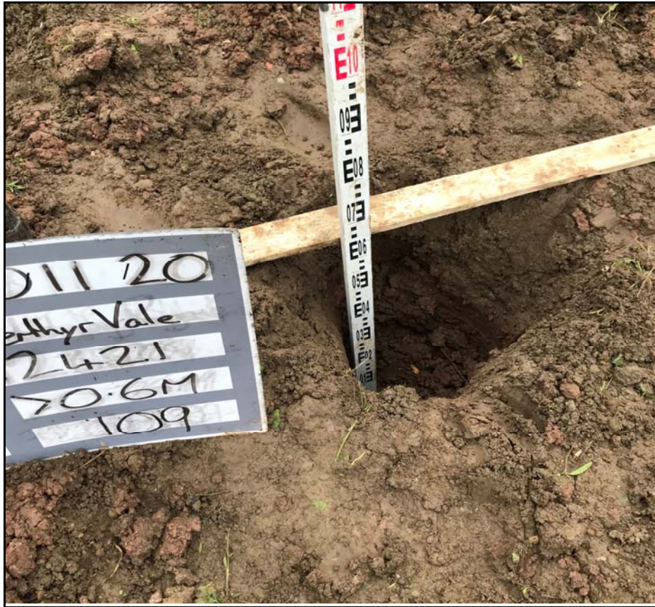
Plot 109 Showing Excavation Trial Pit
