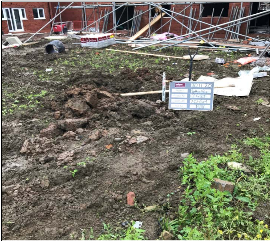
Plot 118 Showing Capping Depth Check
