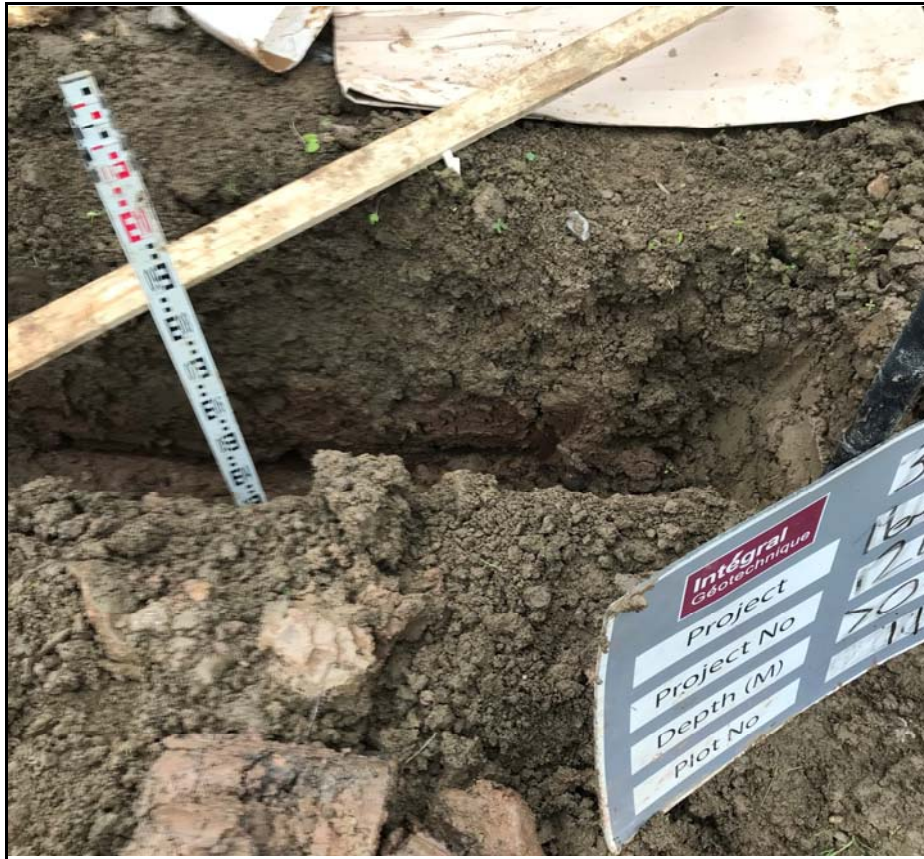
Plot 118 Showing Excavation Trial Pit
