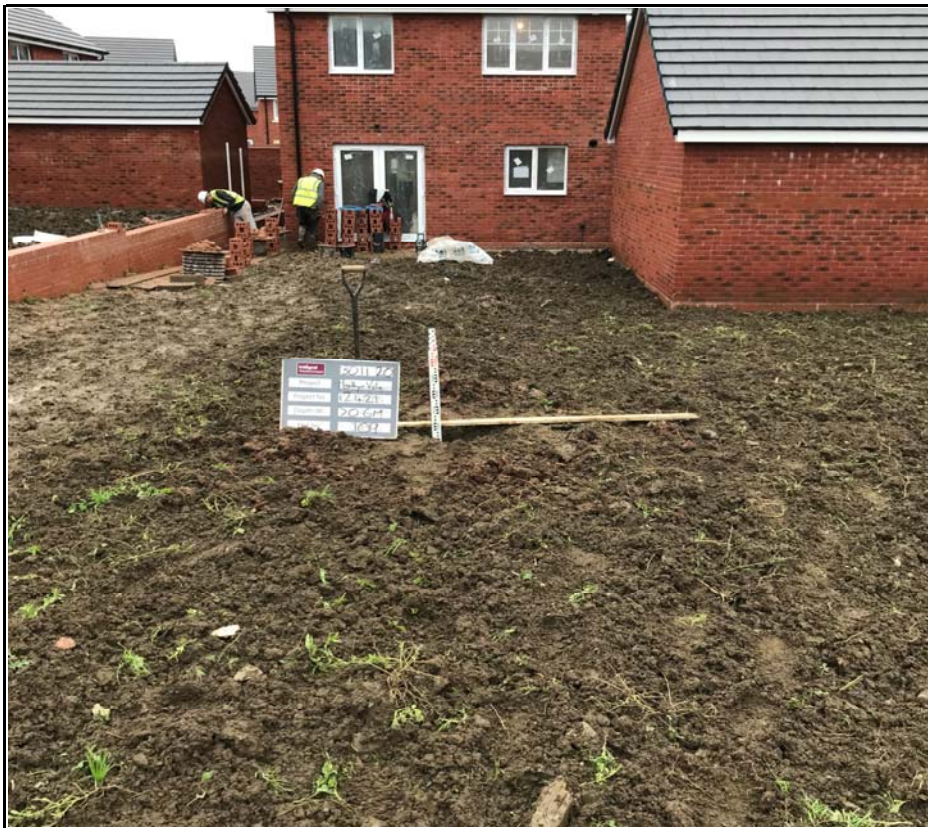
Plot 109 Showing Capping Depth Check
