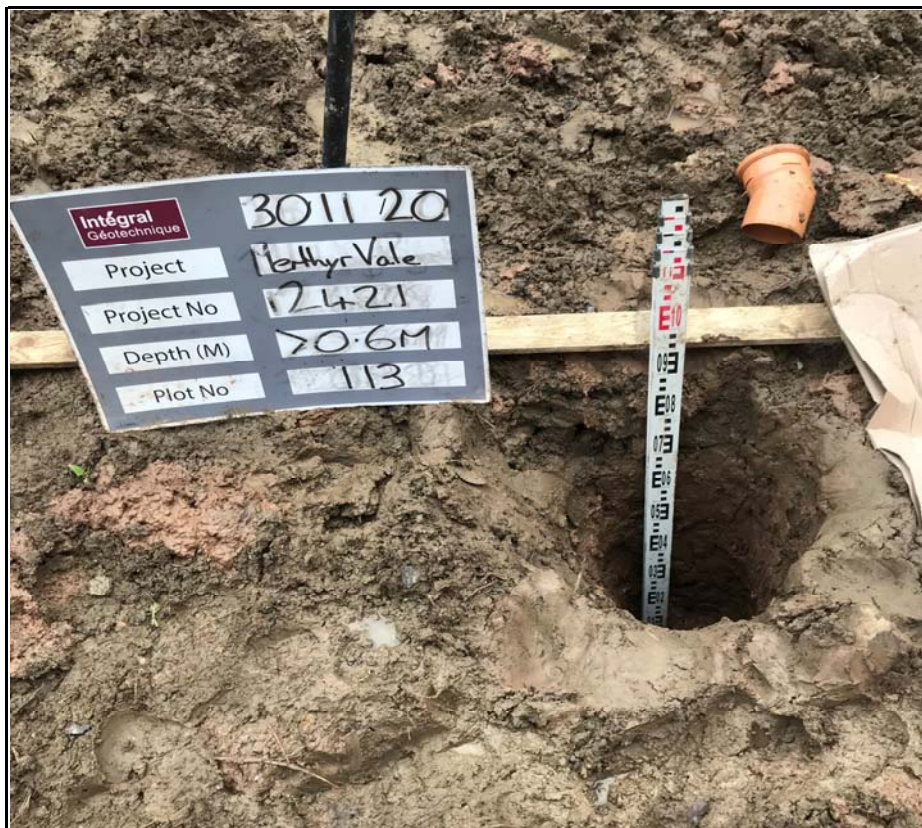
Plot 113 Excavation Trial Pit
