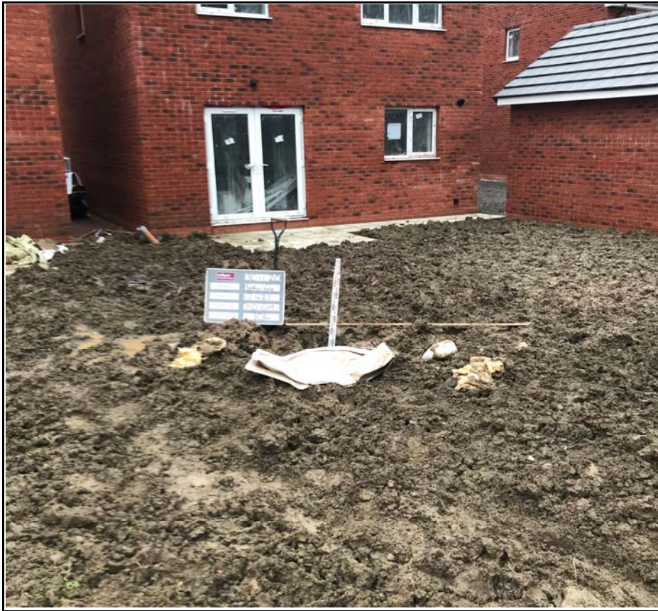
Plot 104 Showing Capping Depth Check
