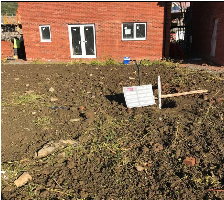
Plot 99 Showing Capping Depth Check
