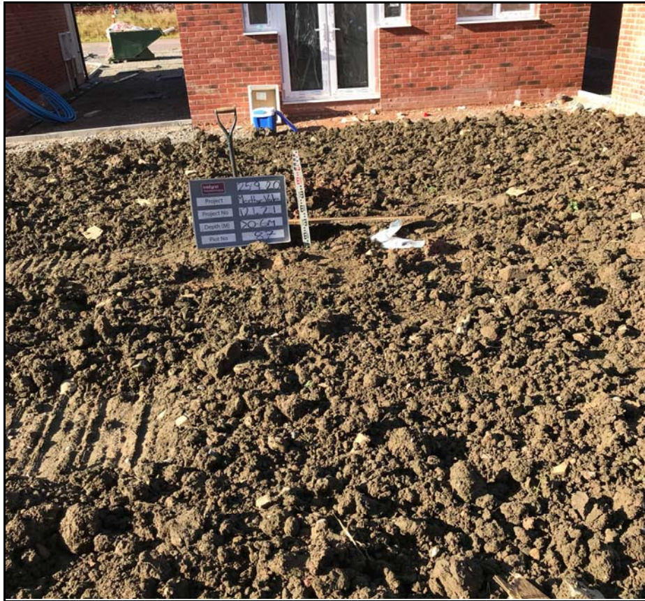
Plot 87 Showing Capping Depth Check
