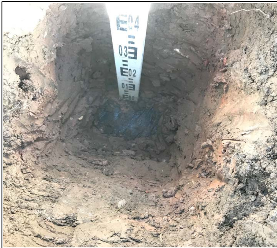
Plot 99 Showing Membrane Placement
