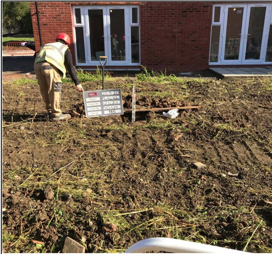
Plot 95 Showing Capping Depth Check
