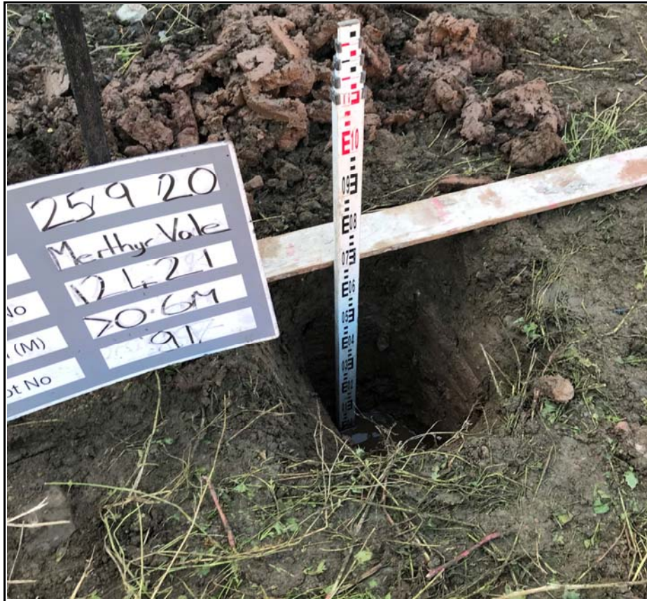
Plot 91 Showing Excavation Trial Pit
