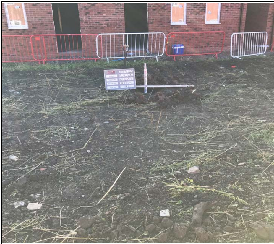
Plot 91 Showing Capping Depth Check
