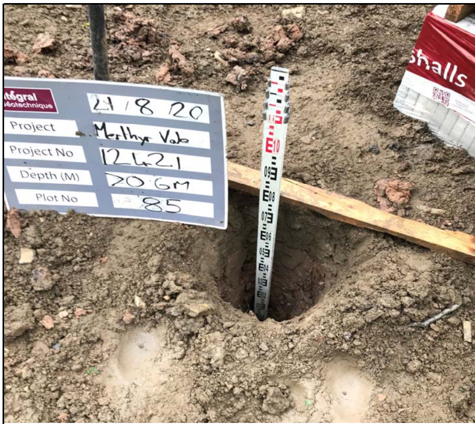
Plot 85 Excavation Trial Pit
