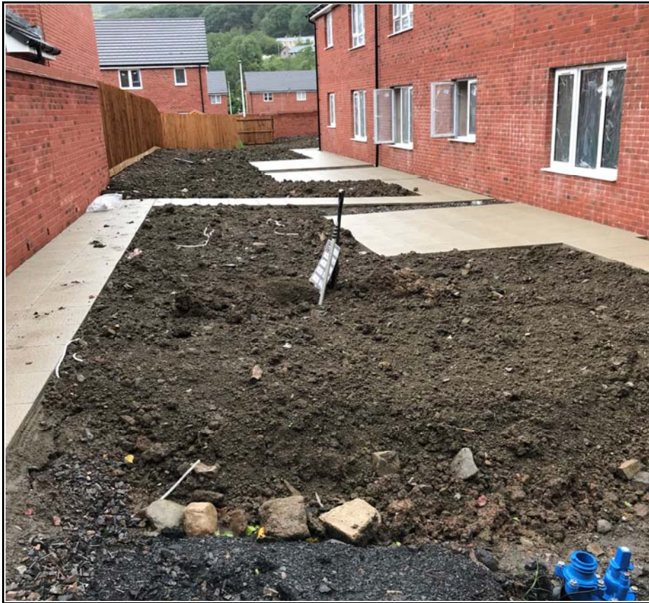
Plot 78 Showing Capping Depth Check
