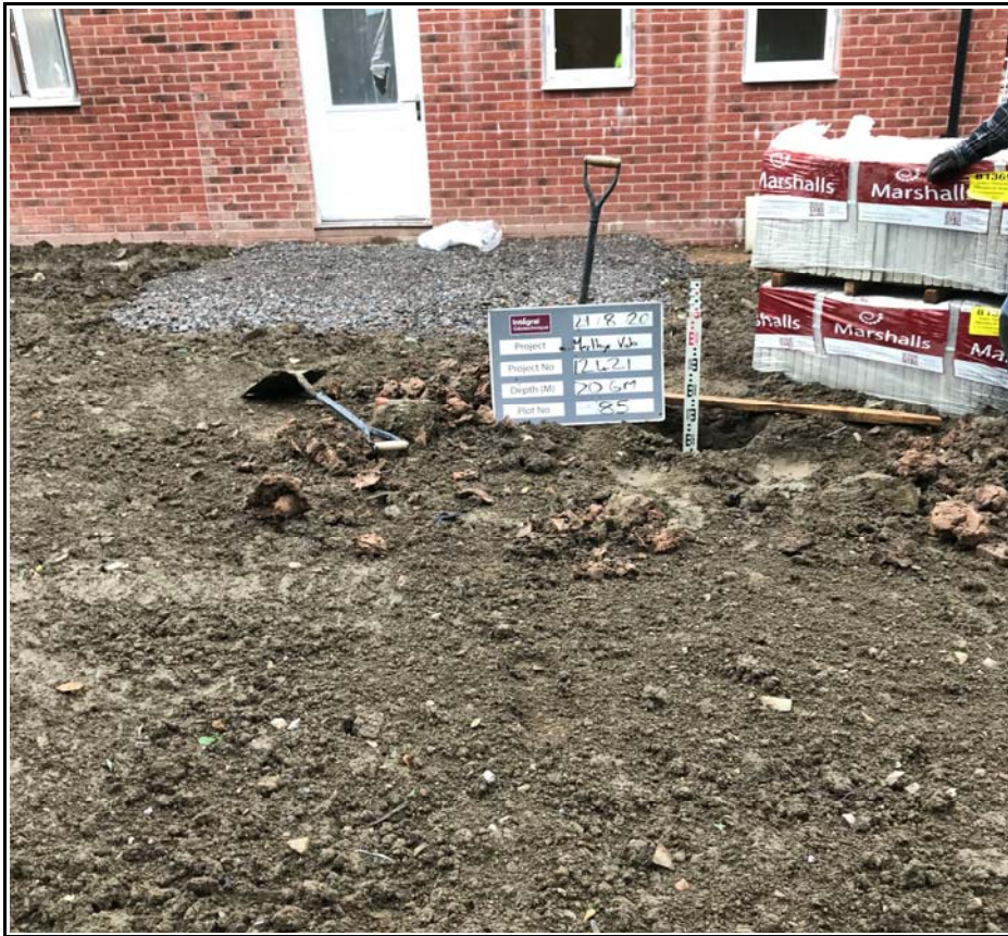
Plot 85 Showing Capping Depth Check
