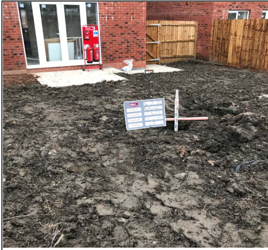
Plot 61 Showing Capping Depth
