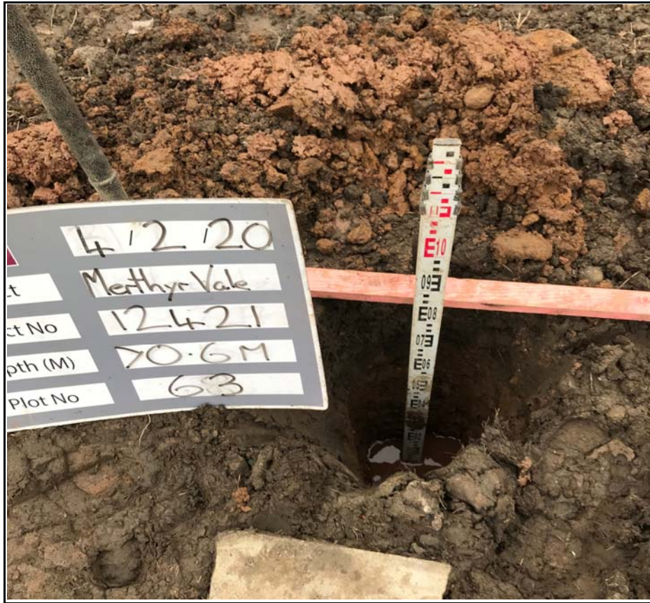
Plot 64 Excavation Pit with Membrane at Base of Soils
