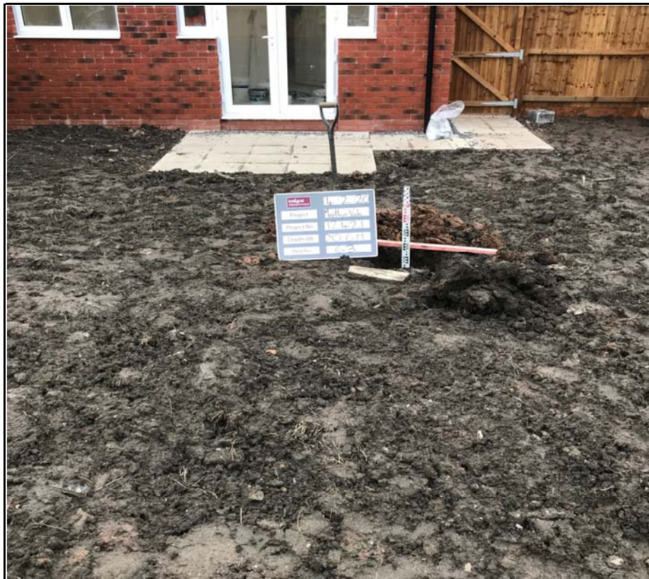
Plot 63 Capping Depth Check
