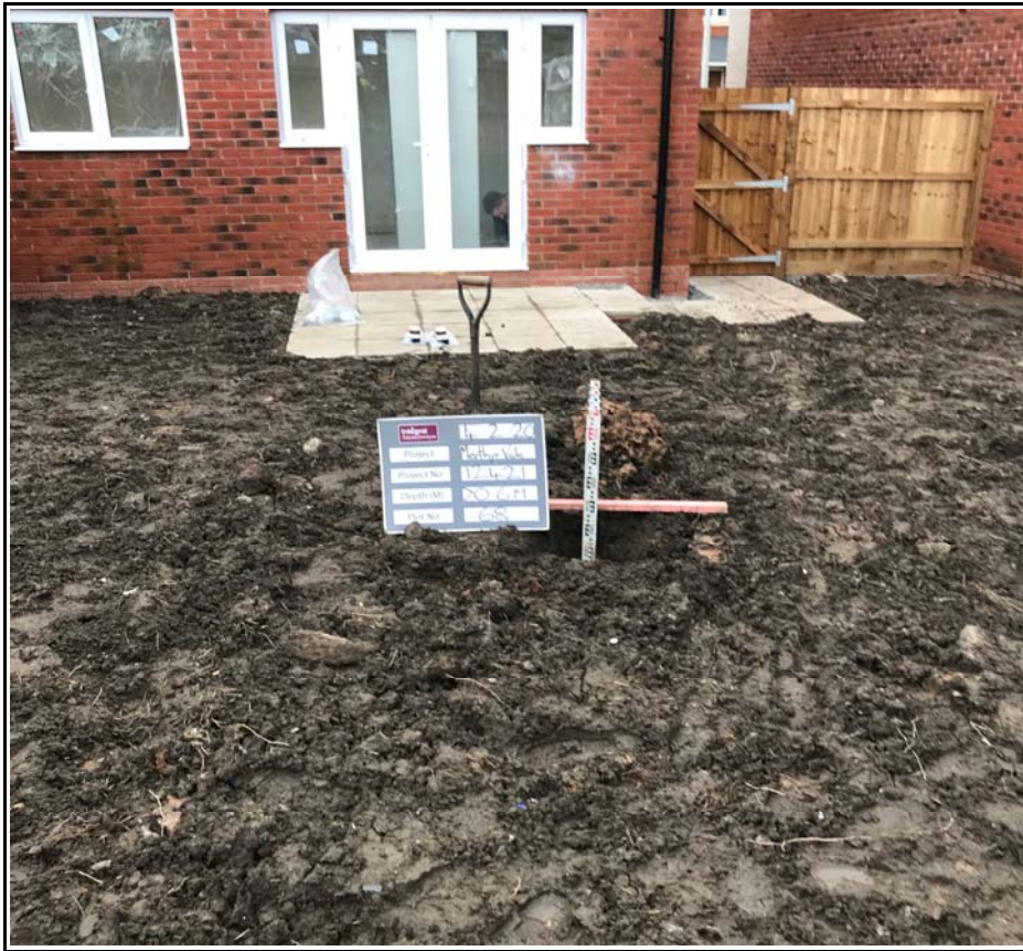
Plot 68 Showing Capping Depth
