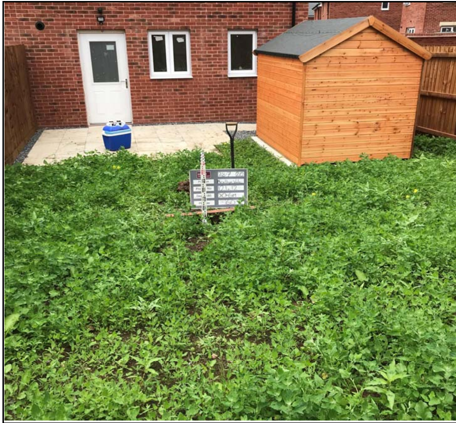
Plot 60 Showing Capping Depth Check
