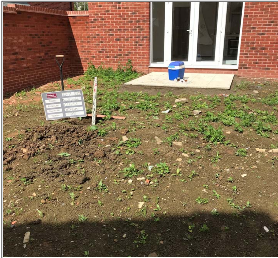
Plot 73 Showing Capping Depth
