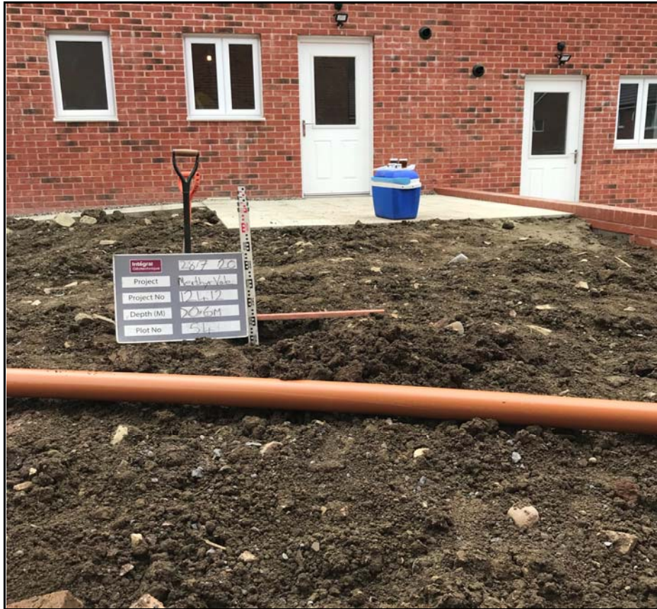
Plot 54 Showing Capping Depth
