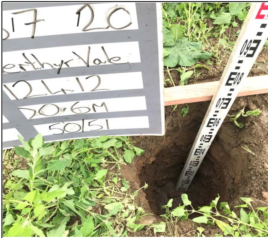
Plot 50/51 Excavation Trial Pit
