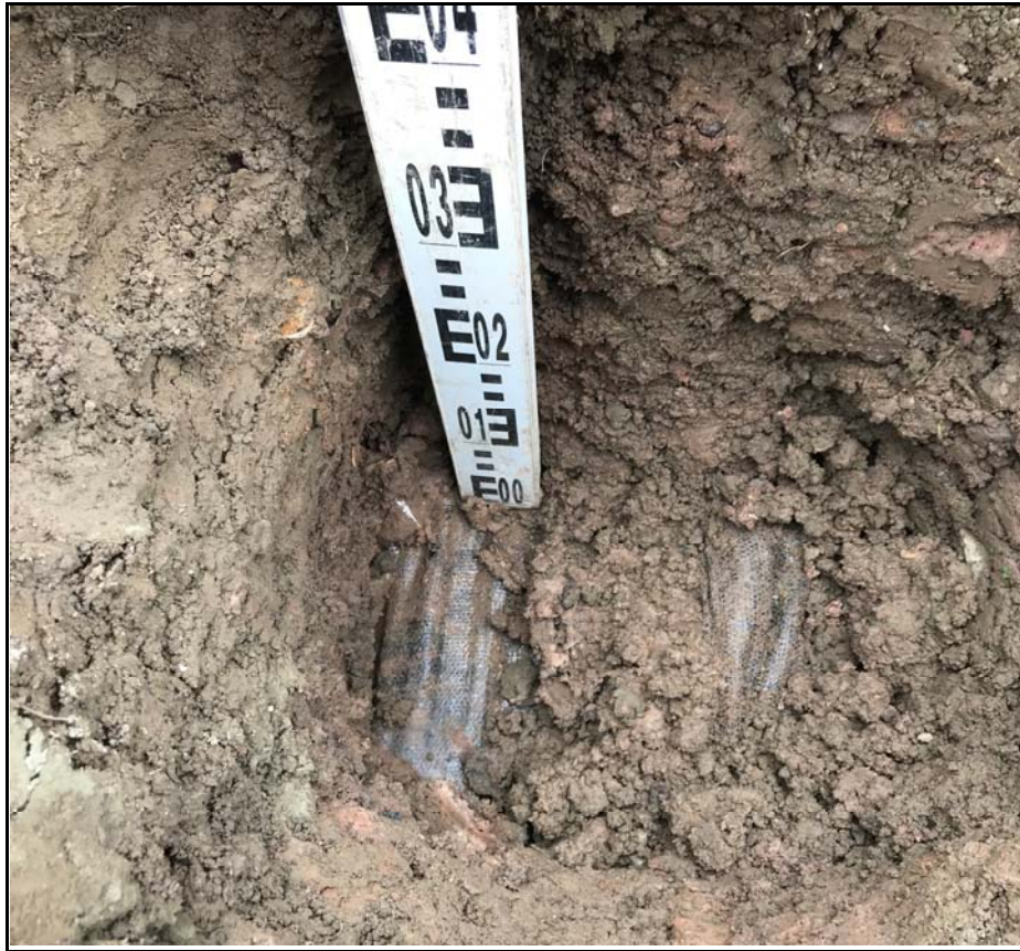
Plot 54 Showing Membrane At Base
