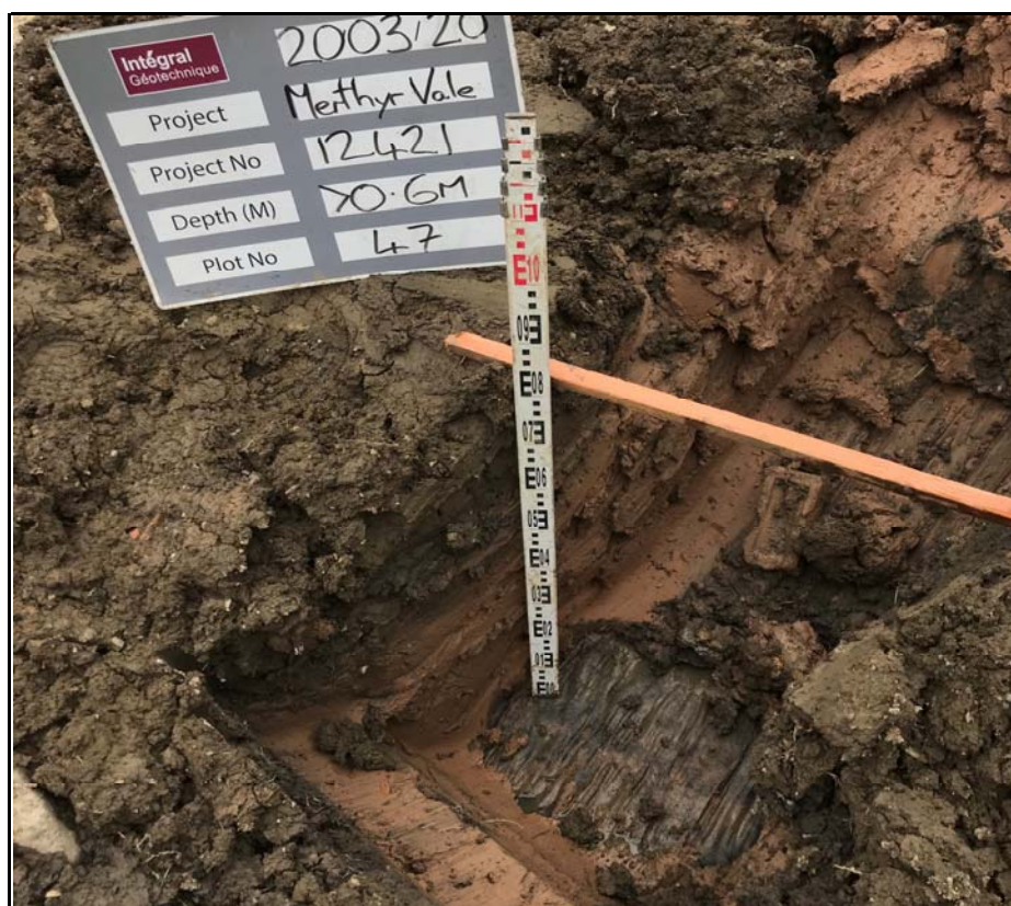
Plot 47 Excavation Pit with Membrane at Base of Soils
