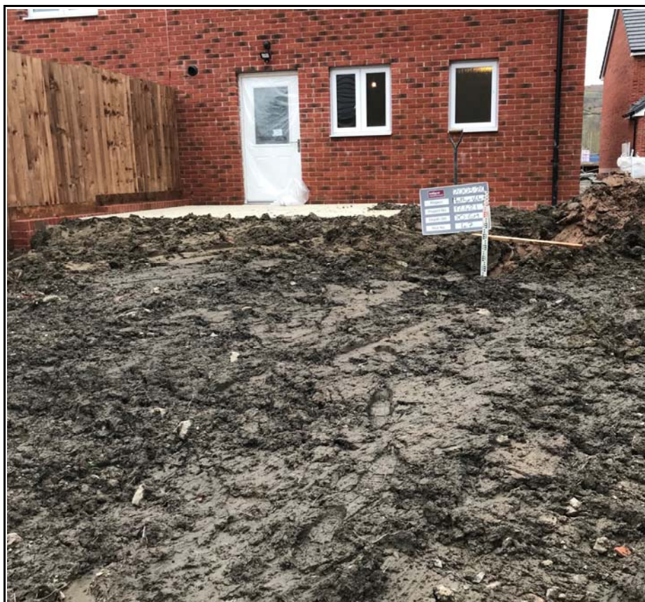
Plot 47 Showing Capping Depth
