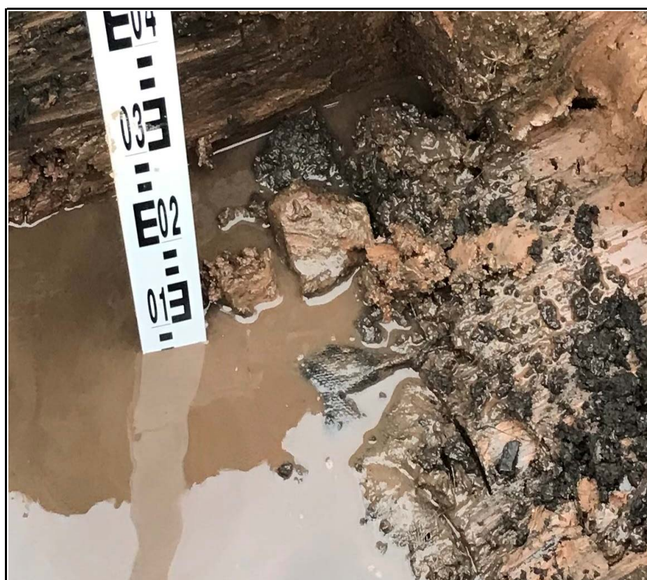
Plot 34 Membrane Presence Through Water Ingress
