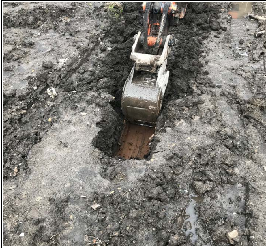
Plot 34 Topsoil And Subsoil Exposure
