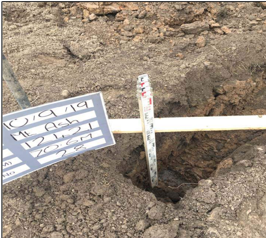
Plot 28 Excavation Trial Pit
