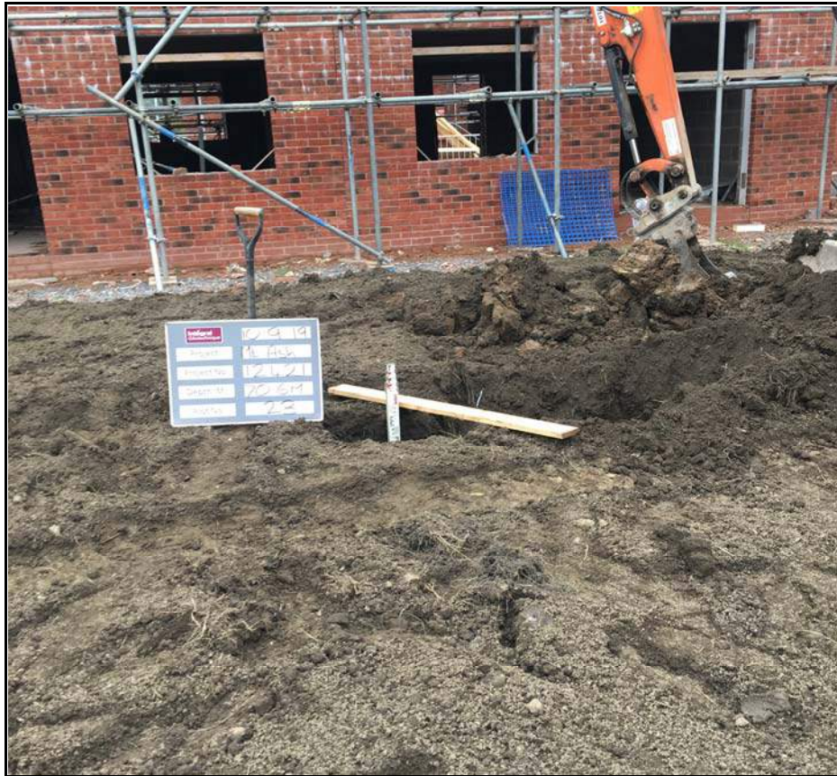
Plot 23 Capping Depth Check
