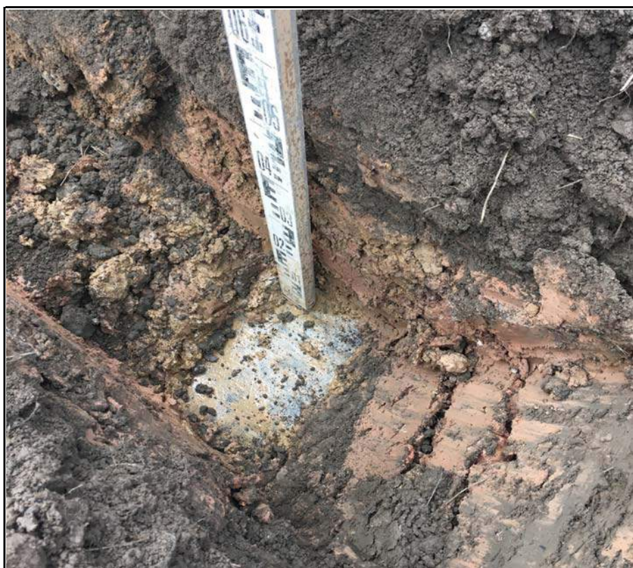
Plot 25 Membrane at Base of Capping Soils
