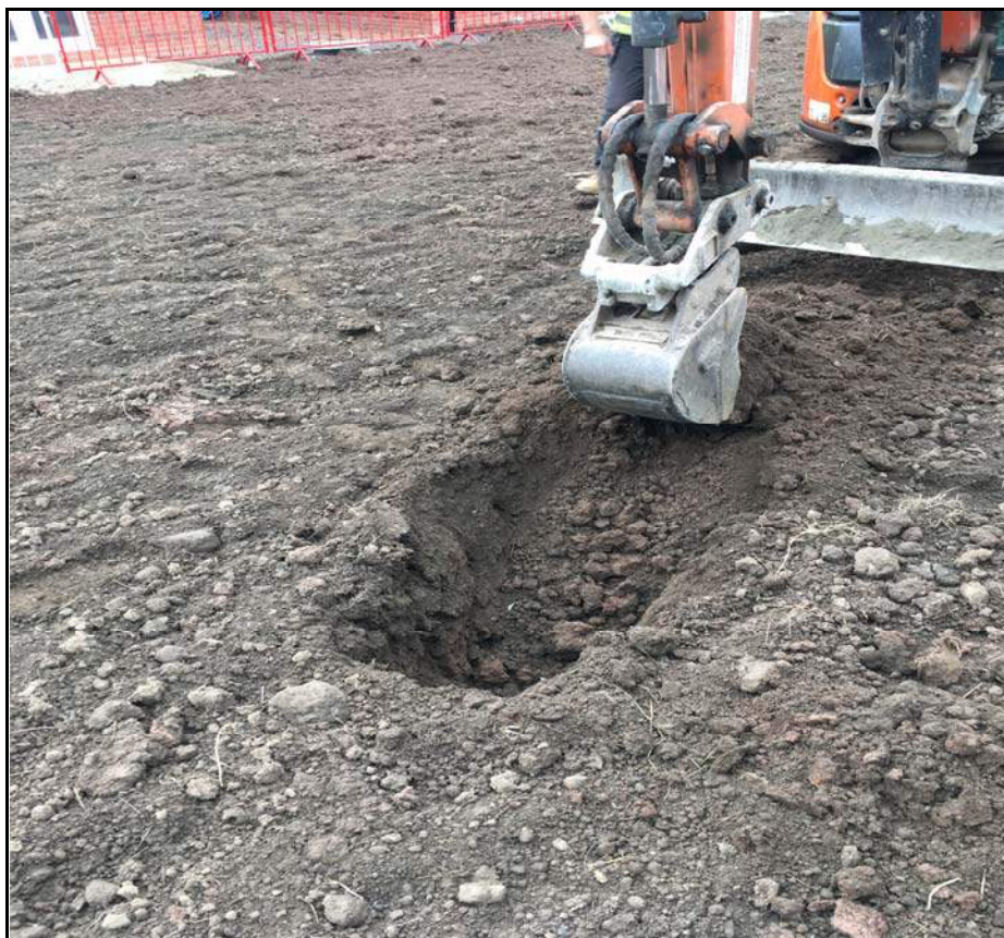
Plot 31 Topsoil And Subsoil Exposure
