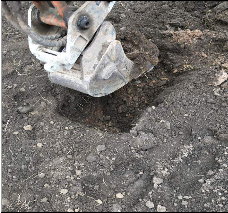
Plot 16 Topsoil And Subsoil Exposure
