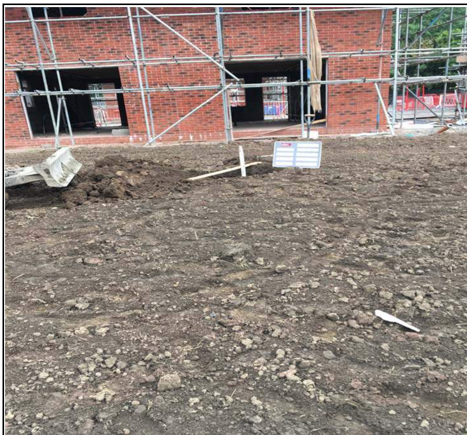
Plot 31 Capping Depth Check
