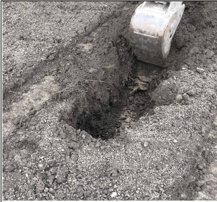
Plot 23 Topsoil And Subsoil Exposure
