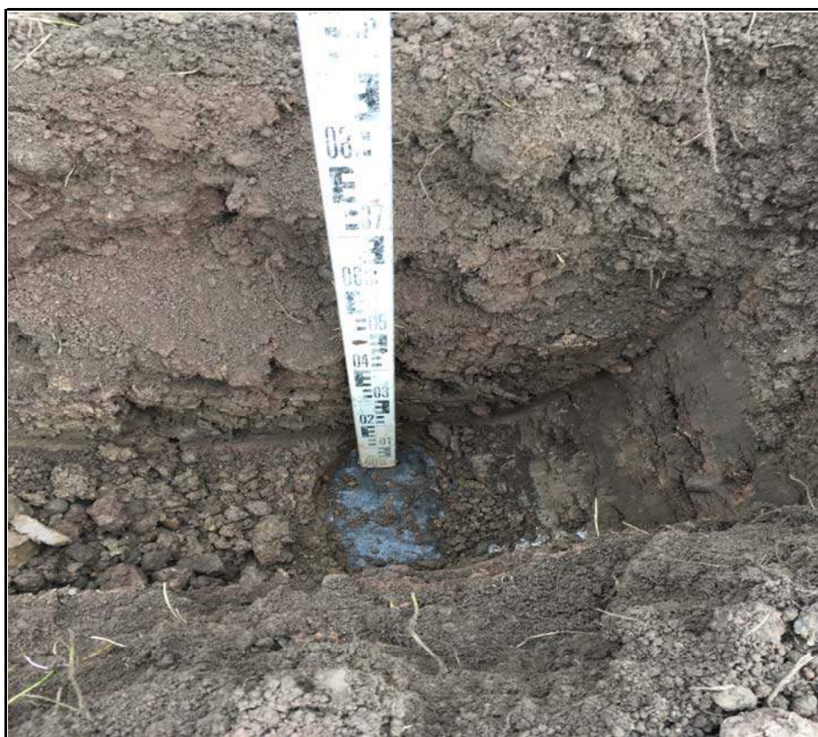
Plot 31 Membrane at Base of Capping Soils
