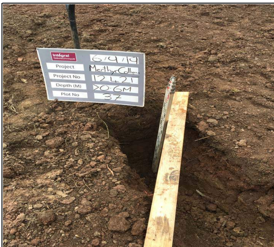
Plot 37 Excavation Trial Pit
