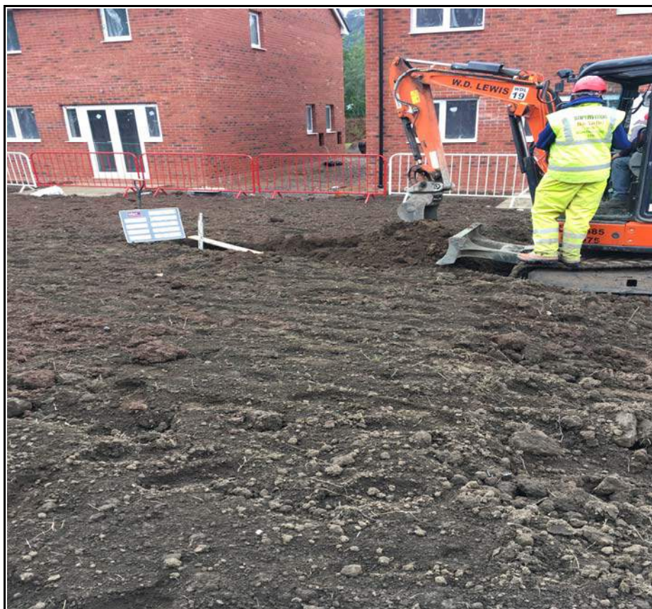
Plot 37 Capping Depth Check
