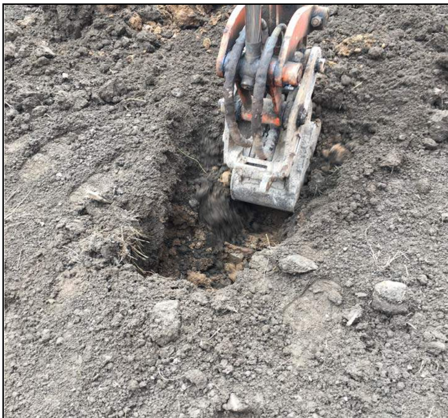
Plot 25 Topsoil And Subsoil Exposure
