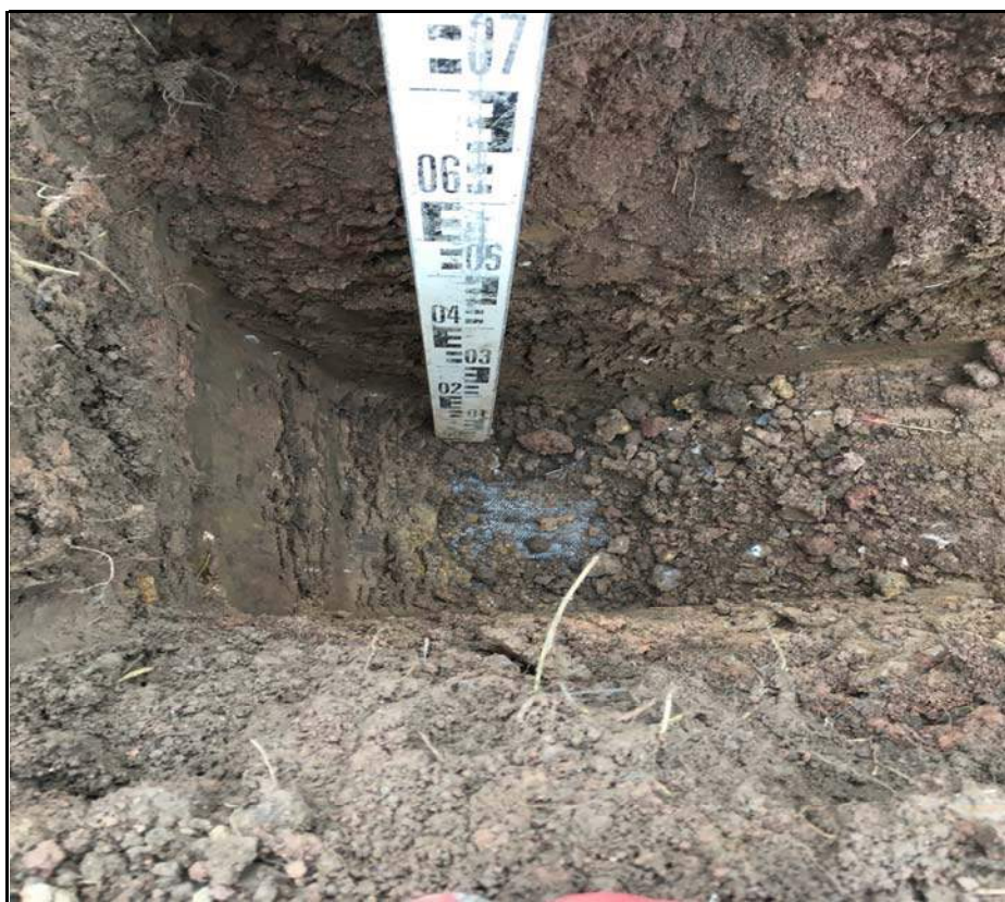
Plot 37 Membrane at Base of Capping Soils
