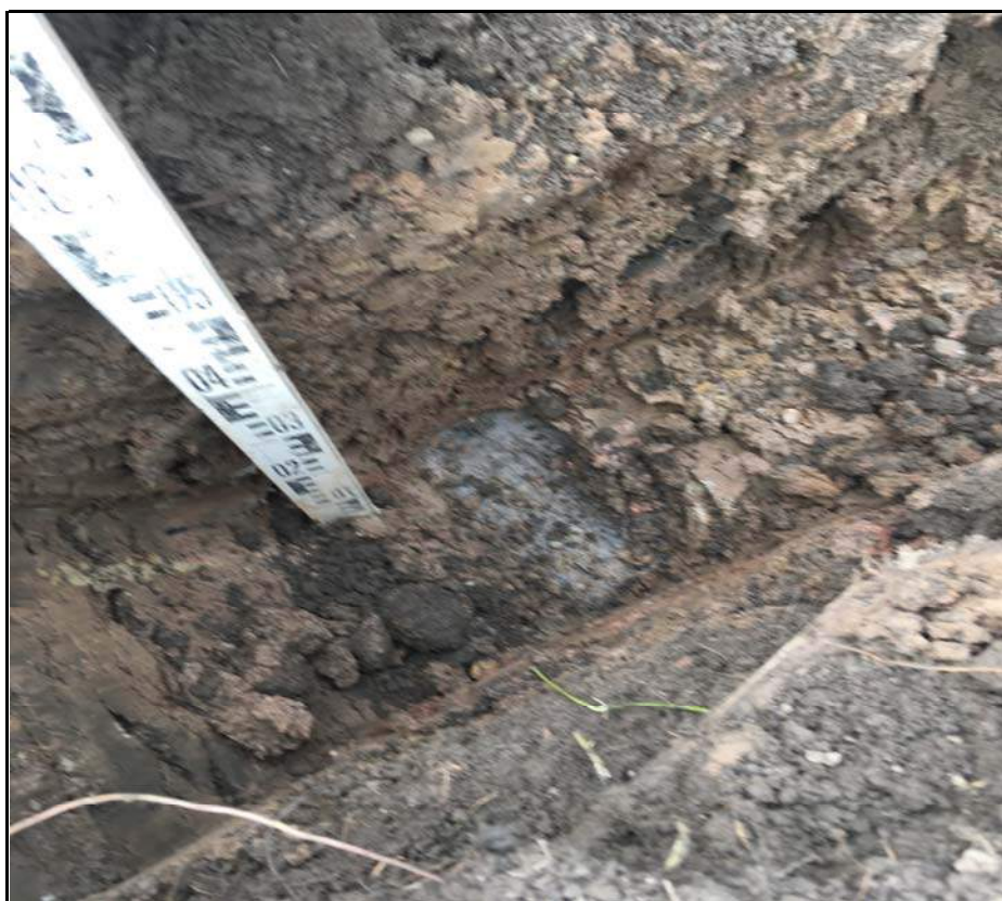
Plot 28 Membrane at Base of Capping Soils
