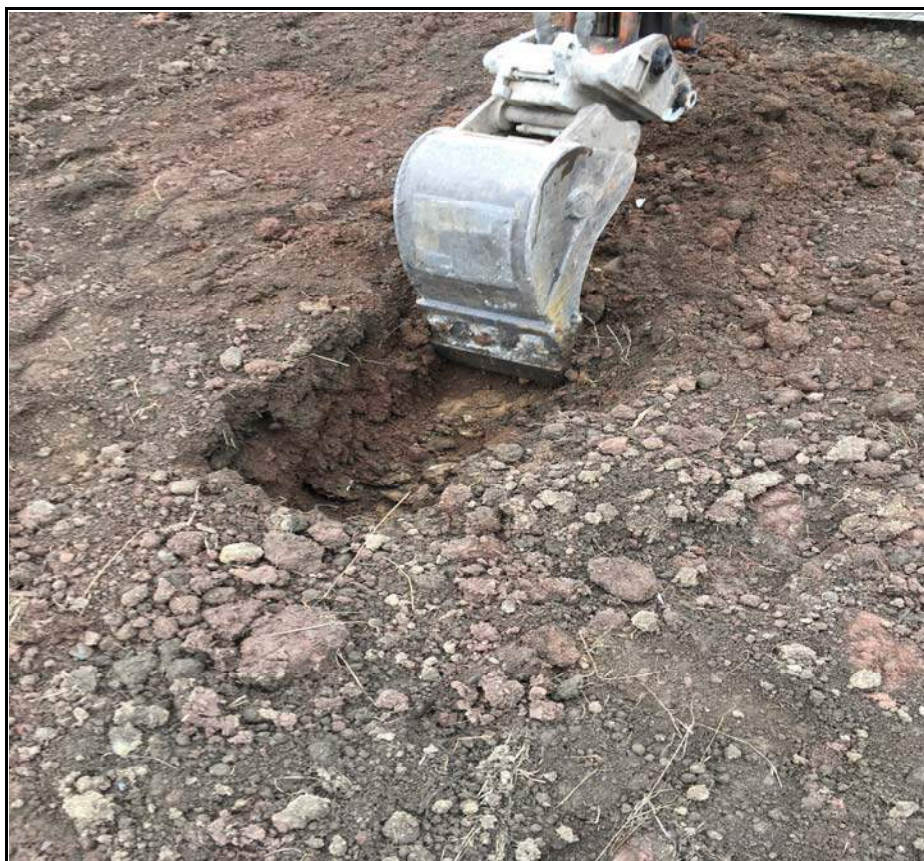
Plot 37 Topsoil And Subsoil Exposure
