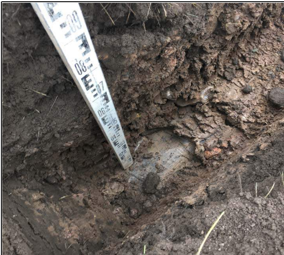
Plot 23 Membrane at Base of Capping Soils
