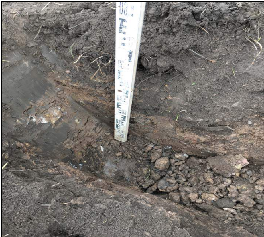
Plot 16 Membrane at Base of Capping Soils
