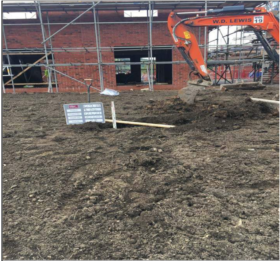
Plot 28 Capping Depth Check
