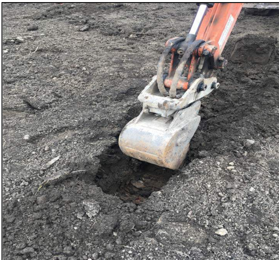
Plot 28 Topsoil And Subsoil Exposure
