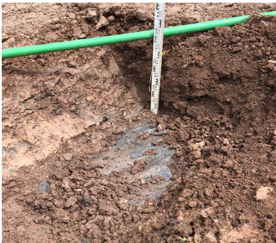
Plot 10 Showing Membrane Placed at Base of Capping
