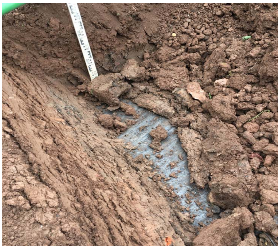
Plot 7 Showing Membrane Placed at Base of Capping
