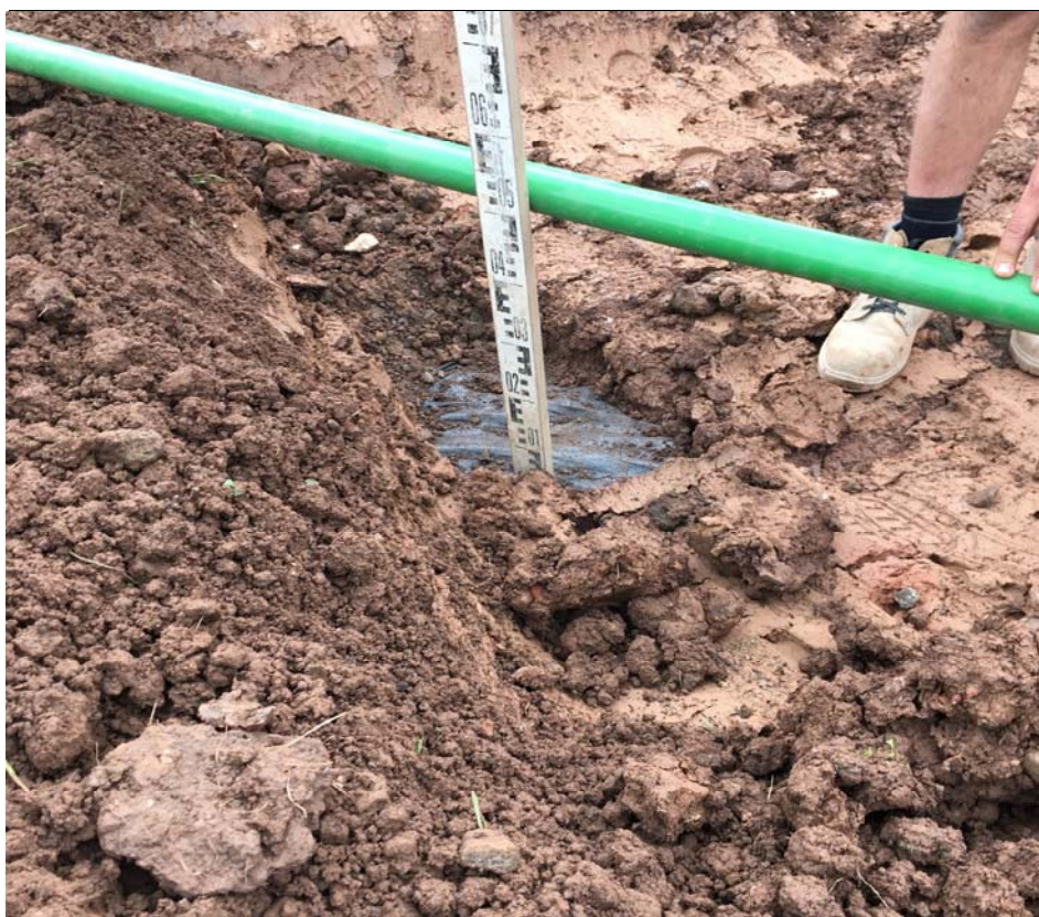
Plot 14 Showing Membrane Placed at Base of Capping
