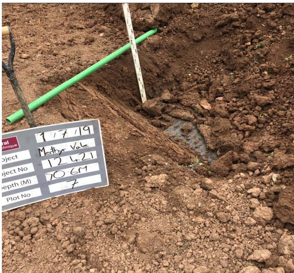
Plot 7 Excavation Pit
