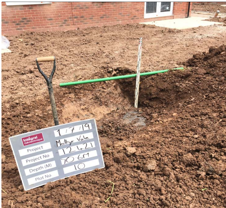
Plot 10 Excavation Pit
