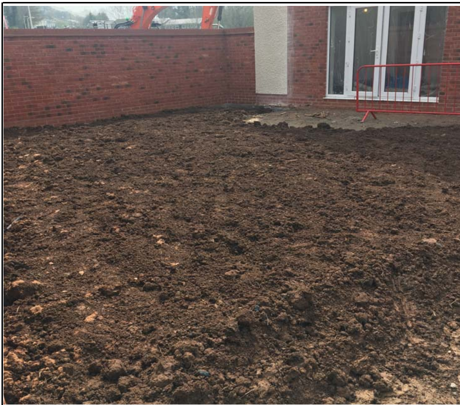
Plot 3 Capping Depth Check
