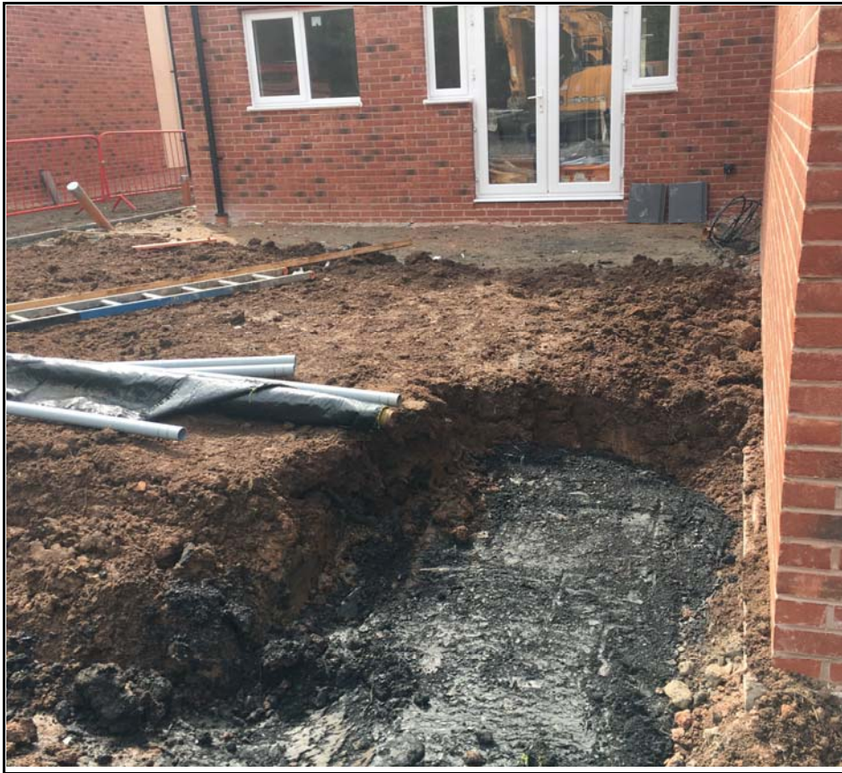
Plot 2 Showing Infilled Garden Area
