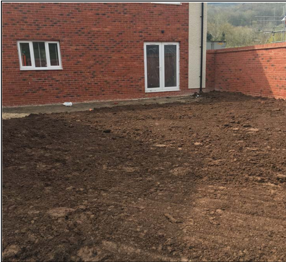
Plot 1 Showing Infilled Garden Area
