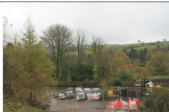
View down onto access verge from site
