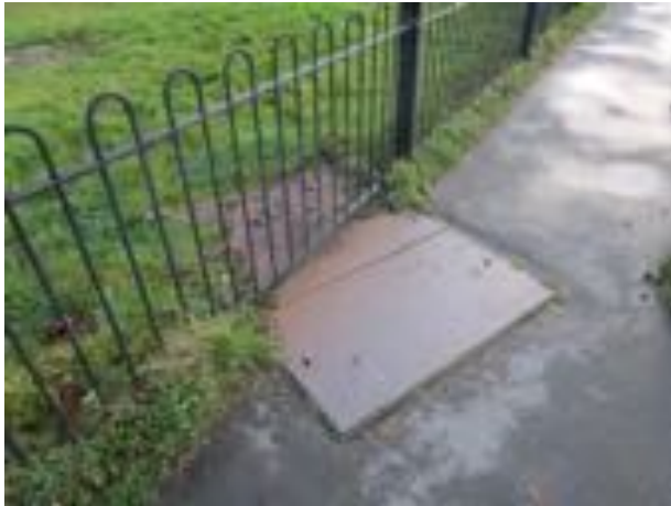
Photo 5 – Metal covers over Welsh Water asset – part on Pant Rd footway, will not form part of the site
