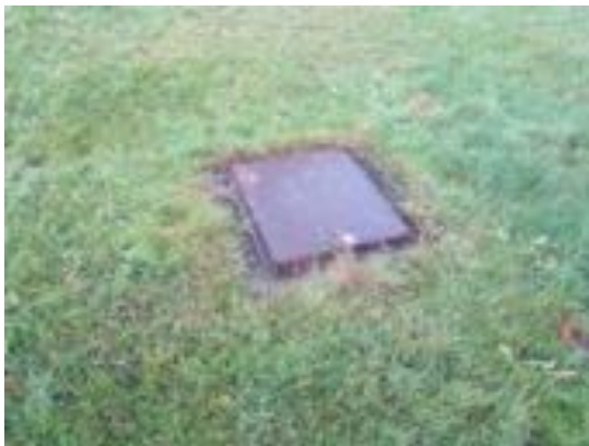
Photo 3 – Metal cover over Welsh Water asset within the proposed site
