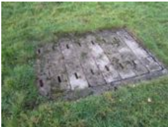
Photo 2 – Slatted concrete cover over Welsh Water asset within the proposed site
