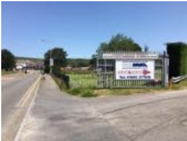
Photo 9 - main entrance from Pant Road
