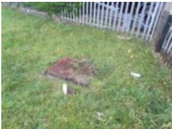
Photo 4 – Metal cover over Welsh Water asset to the western edge of the site
