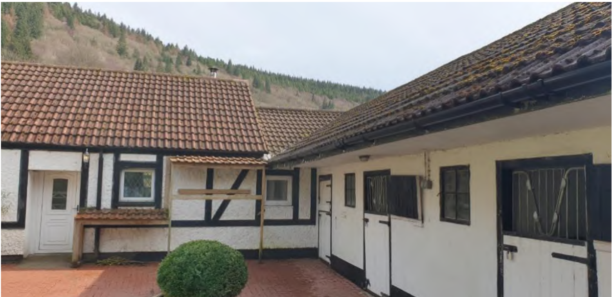
2) North elevation adjoined to farmhouse
