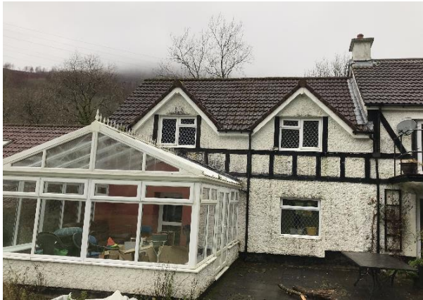
Photo 11: Western Elevation Lean-to With Gaps Under Ends of Tiles
