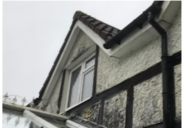
Photo 12: Western Elevation Lean-to With Gaps Under Ends of Tiles
