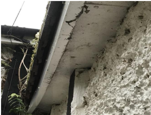
Photo 19: Gap Between Soffit and Tiles
