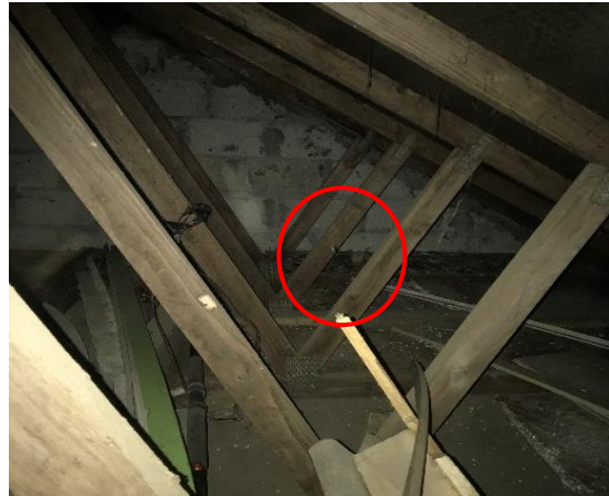
Photo 30: Attic Space Above Void 3 – Nest Location Indicated
