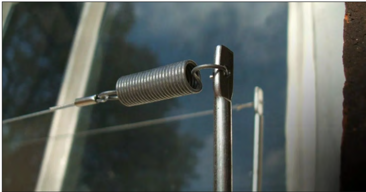
Example: Spring bird wire to top of flex box
