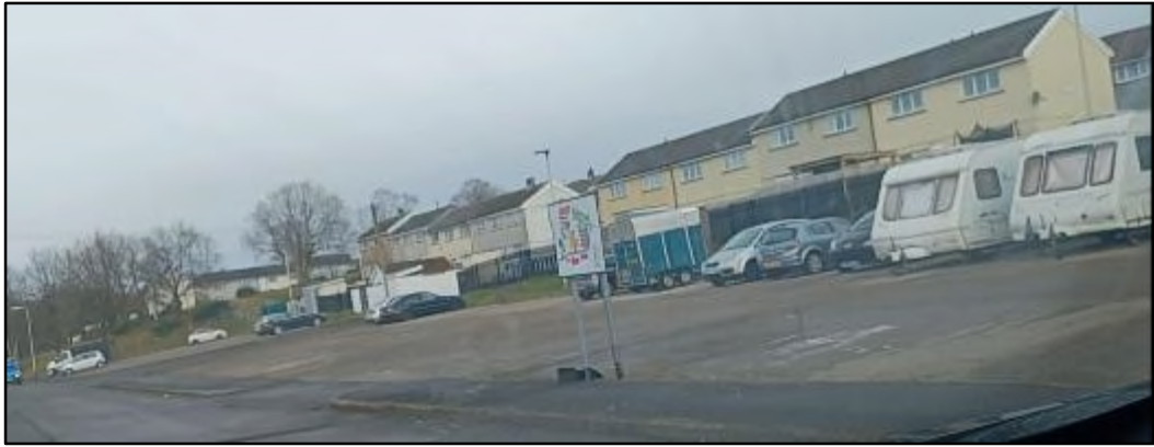
Plate 2.3 Crabapple Close Parking Area – looking north
