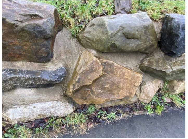
Detail of rock and mortar retaining wall along northern boundary
