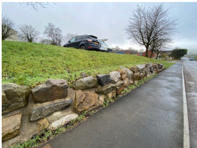
Northern boundary viewing west along Gurnos Ring Road, showing rock and mortar wall
