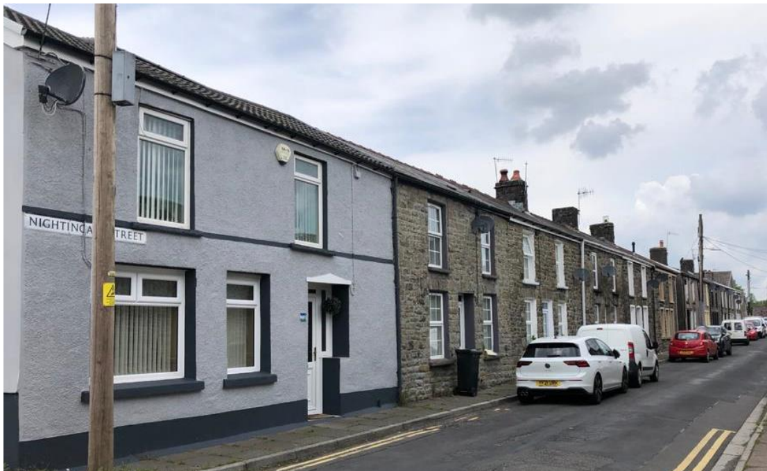
Unsympathetic front extension in terrace and communal walkway to terraced properties
