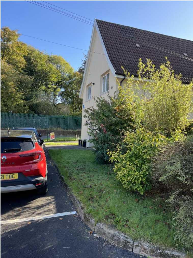
Image of the existing side grass area proposed to be partially removed to form a new paved pathway (Source: DMP photo 2025)
