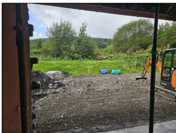
Plate 5 – The works occurring on site.
