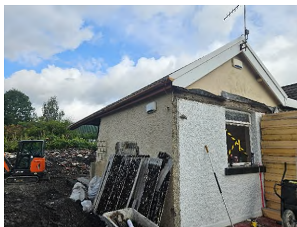
Plate 6 – The plastic soffit and fascia boards.
