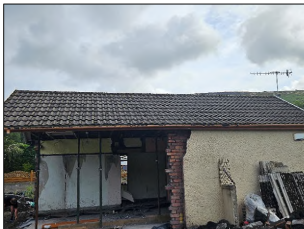
Plate 3 – The roof tiles in good condition.
