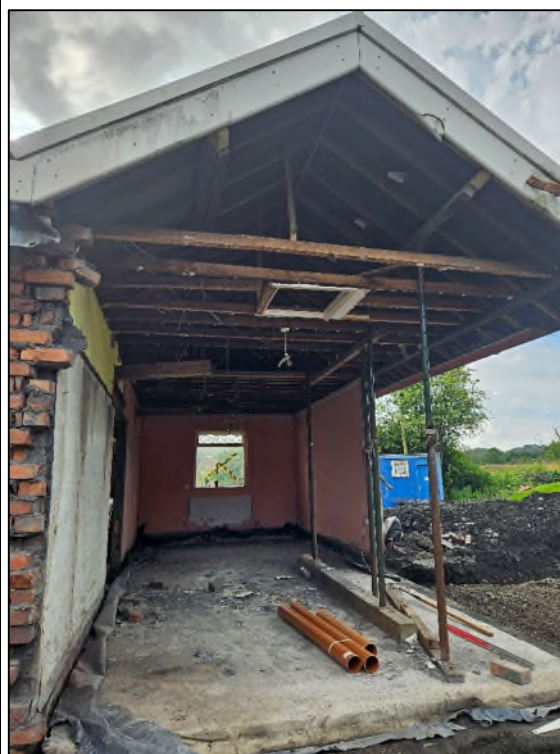
Plate 2 - The two outer walls being removed.
