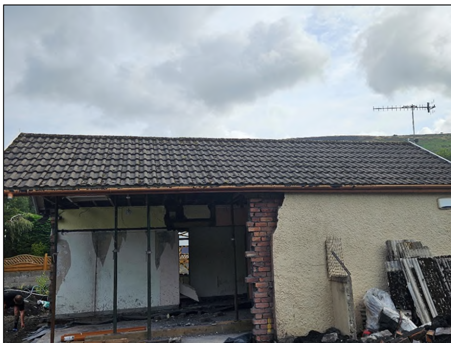
Figure 5: The building from the South side.
