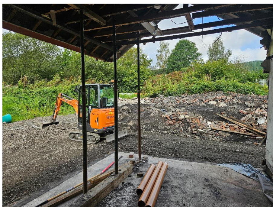
Figure 4 - The habitat surrounding the site.
