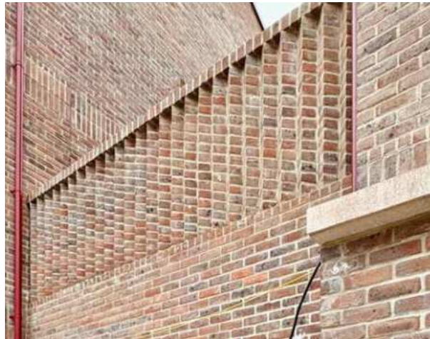
Brickwork detailing to terraces (see 11, on previous page)
