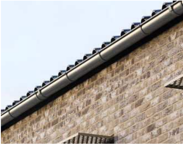
Galvanised steel rainwater goods
