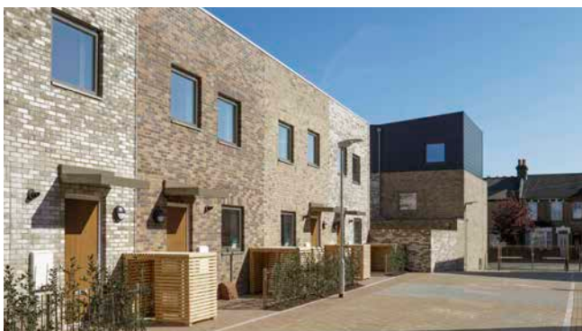
Metal railings & planting with integrated heat pump or bin storage.
