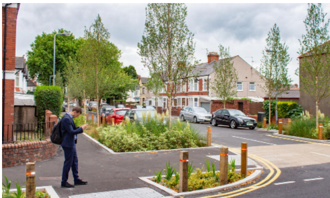
Raised kerbs and timber posts/ knee rails.
