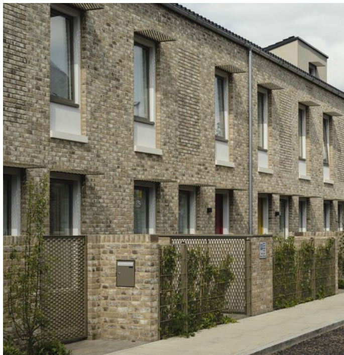
Brick walls & metal fencing with planting.
