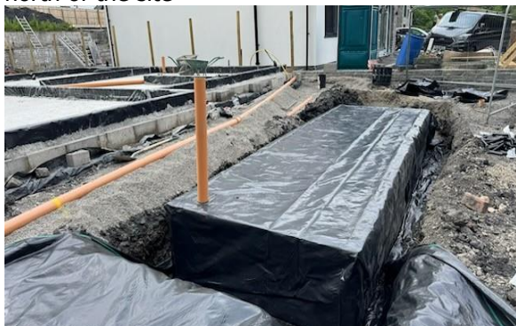
Photo 9: The attenuation within Plot 8 to the north of the site
