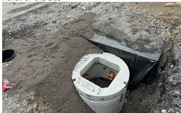
Photo 10: The attenuation within Plot 8 to the north of the site
