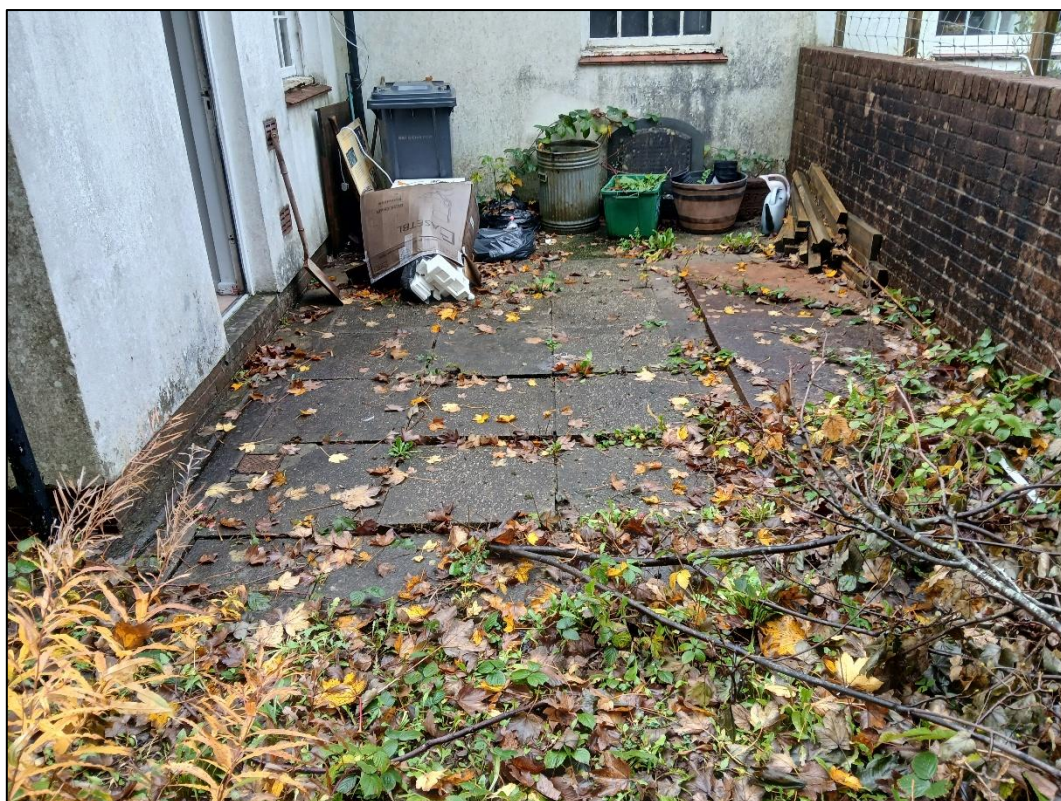
Plate 15. Patio at the rear of No. 4 Chapel Row, looking west-southwest.
