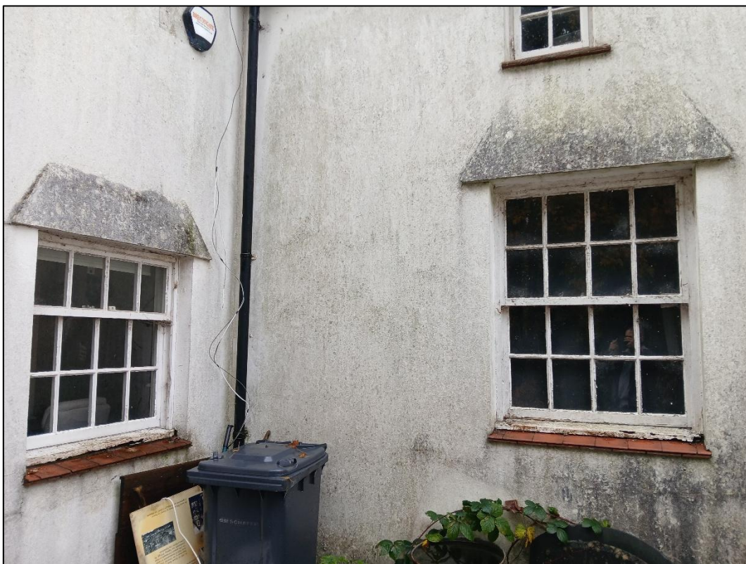
Plate 14. Windows at the rear of No. 4 Chapel Row, showing flared raised hood above each, looking southwest.
