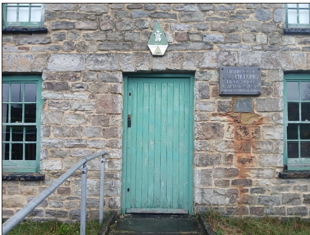
Plate 6. Front door of No. 4 Chapel Row, showing stone and metal plaques, looking east-northeast.
