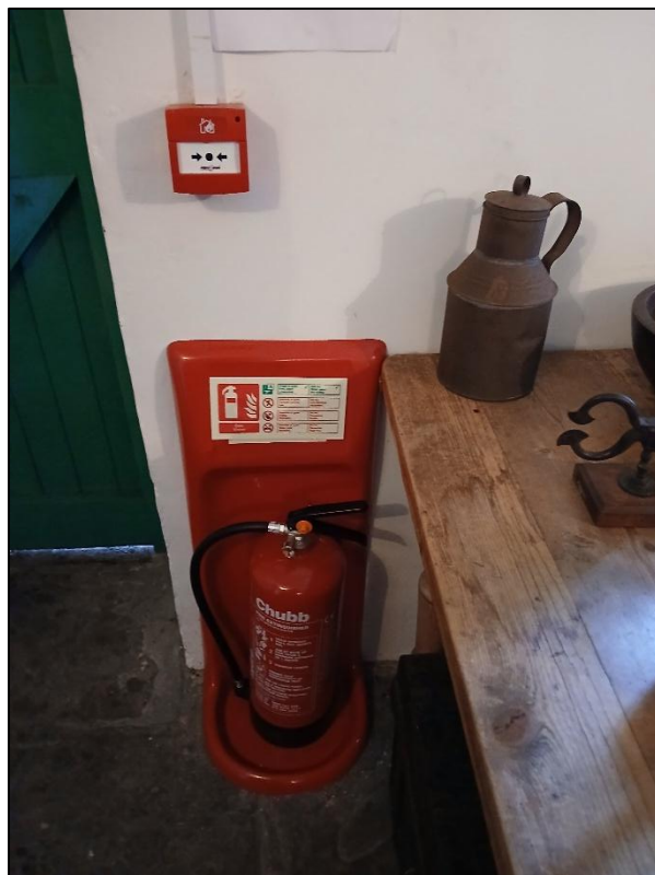
Plate 23. Fire alarm and fire extinguisher seen on the ground floor of No. 4 Chapel Row, looking west-southwest.
