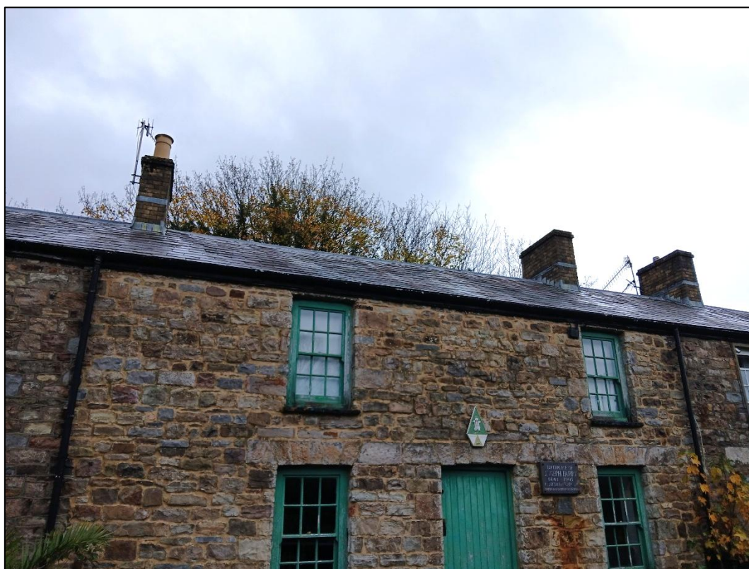
Plate 8. Roof of No. 4 Chapel Row, looking east-northeast.
