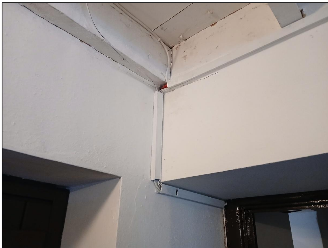
Plate 22. Example of wiring seen on the ground floor of No. 4 Chapel Row, looking east.
