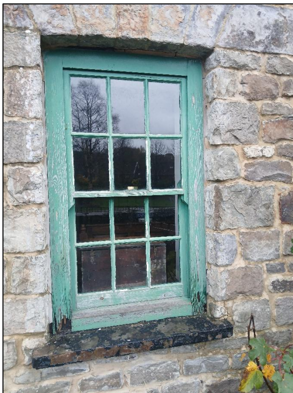
Plate 5. Front right window of No. 4 Chapel Row, looking east-northeast.
