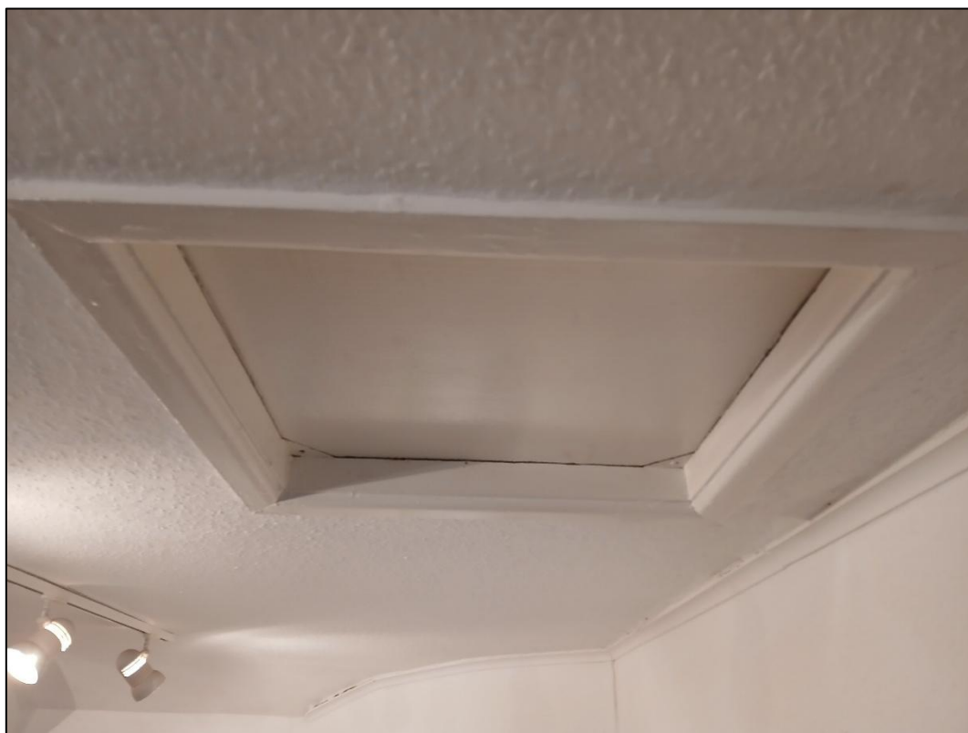
Plate 36. Loft hatch in showroom on first floor of No. 4 Chapel Row, looking west-southwest.
