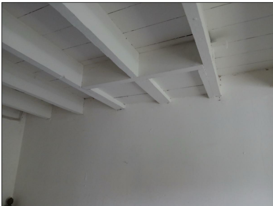
Plate 20. Example of painting ceiling and walls in the ground floor rooms of No. 4 Chapel Row, looking east.
