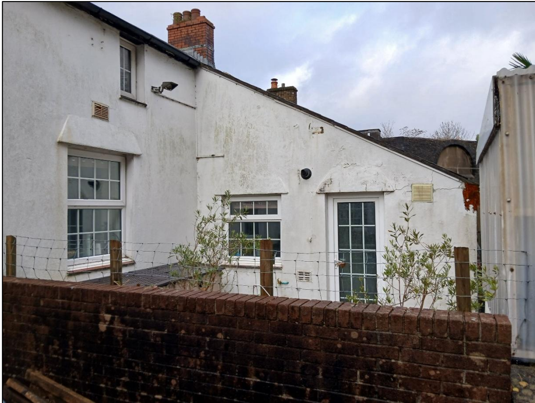
Plate 13. Modern extension to the rear of No. 2 and No. 3 Chapel Row, looking northwest.
