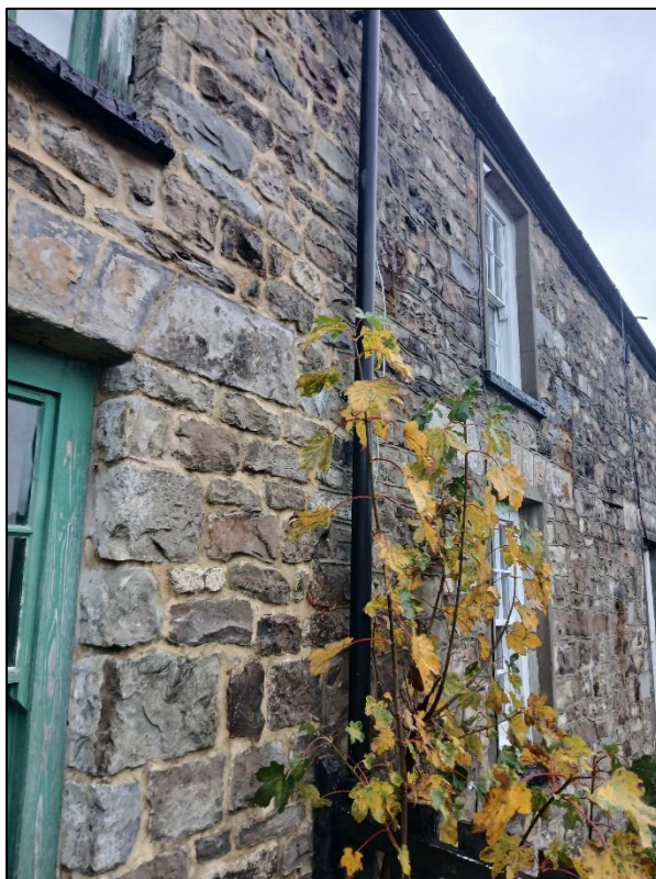
Plate 7. Modern drainpipe and wiring seen at the front of No. 4 Chapel Row, looking east.
