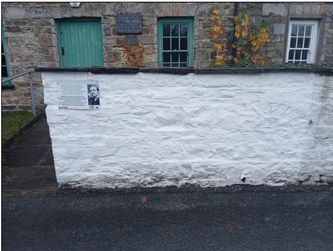
Plate 10. White painted wall, running along the forecourt of cottages on Chapel Row, looking east-northeast.
