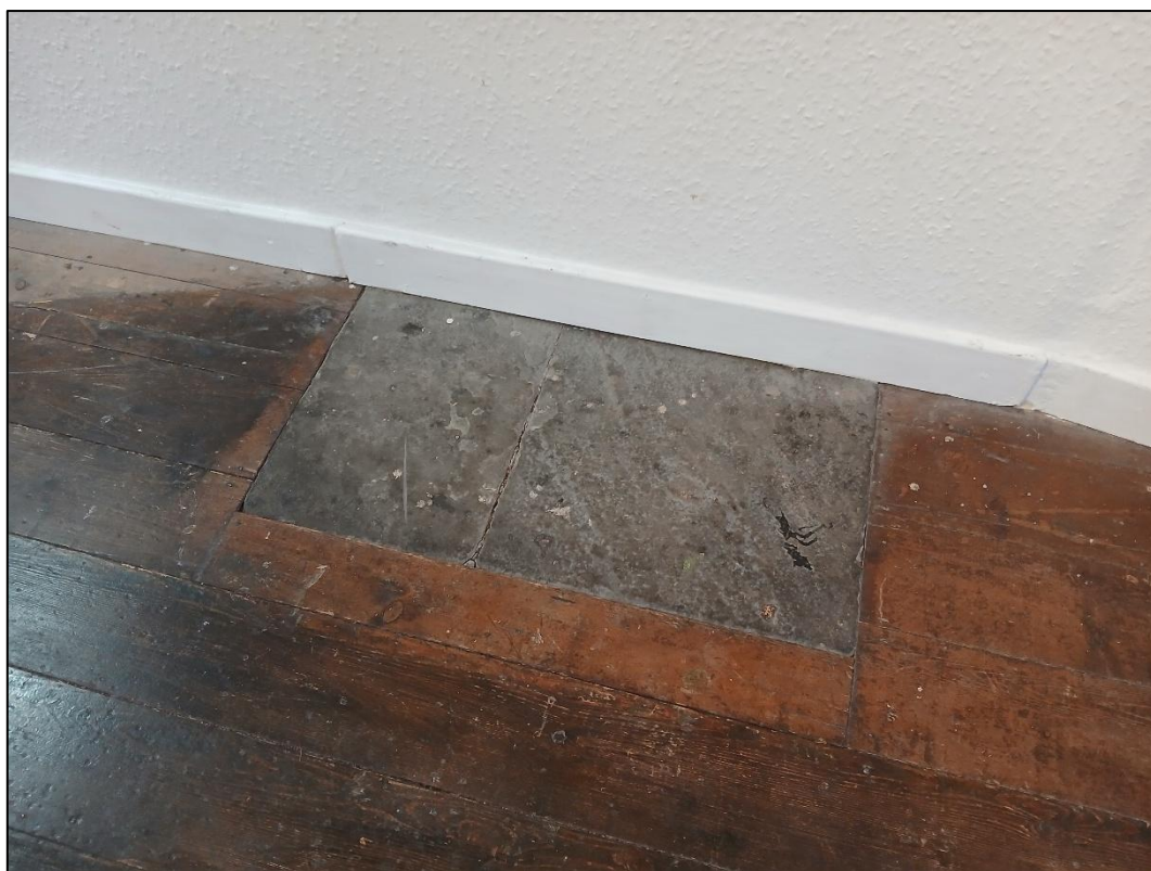
Plate 35. Flagstone indicating the location of a fireplace behind the stud wall in the hallway on the first floor of No. 4 Chapel Row, looking southeast.
