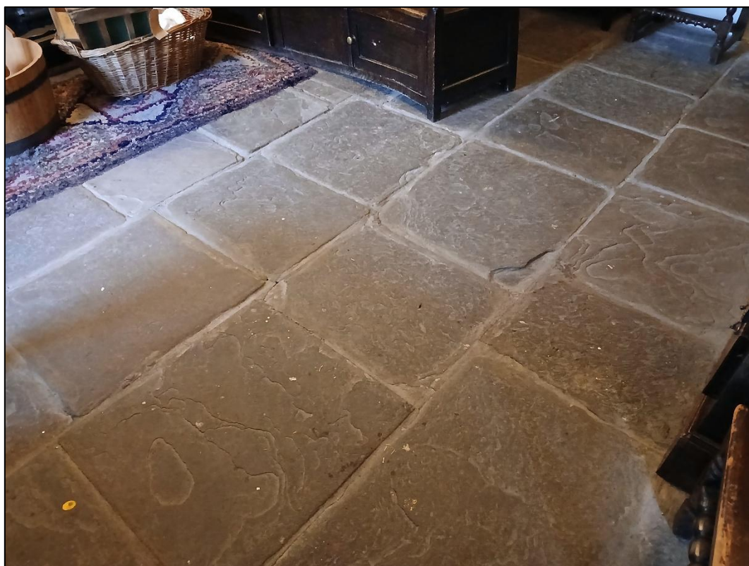
Plate 19. Example of the flagstone floor on the ground floor of No. 4 Chapel Row, looking north.
